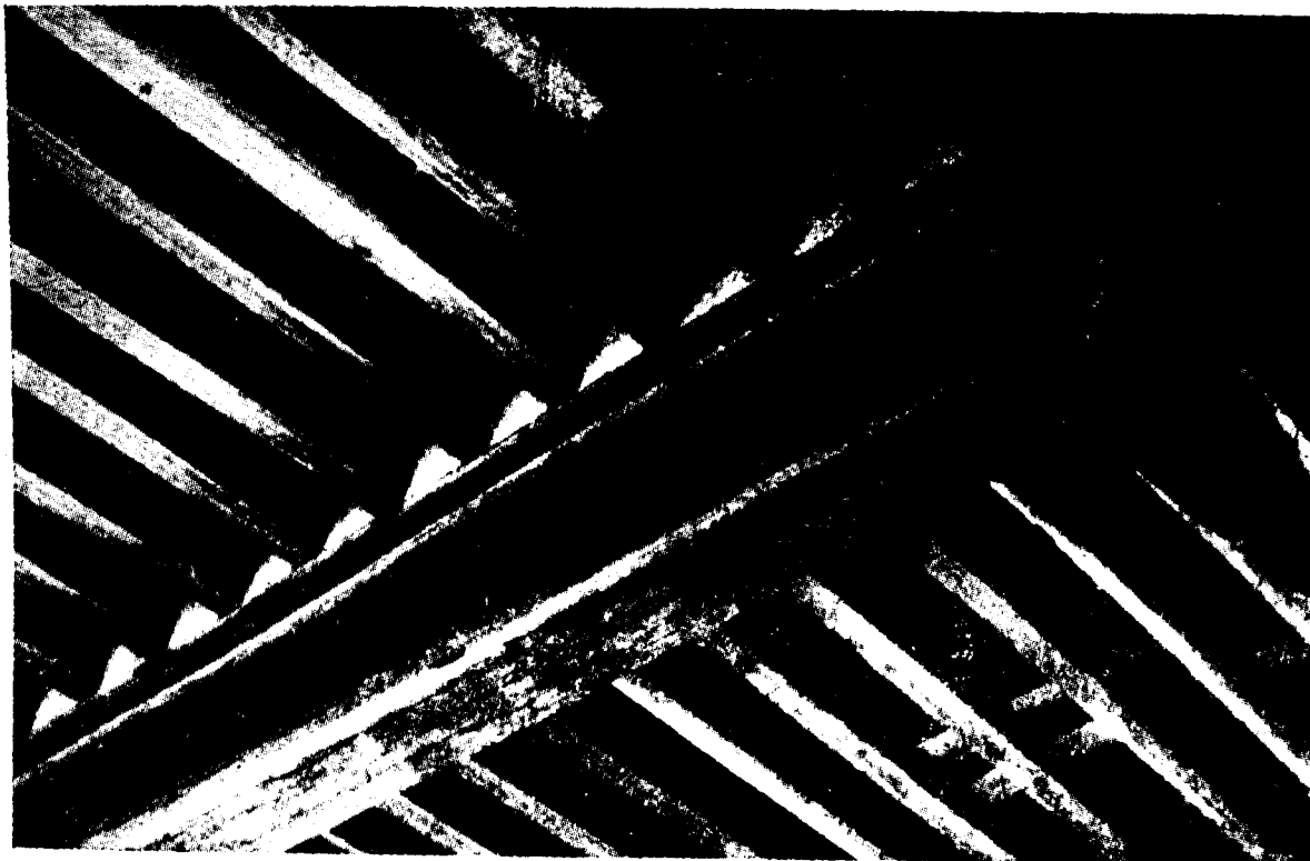
Roof of a pucca house All the beams and linteis are of seasoned wood
