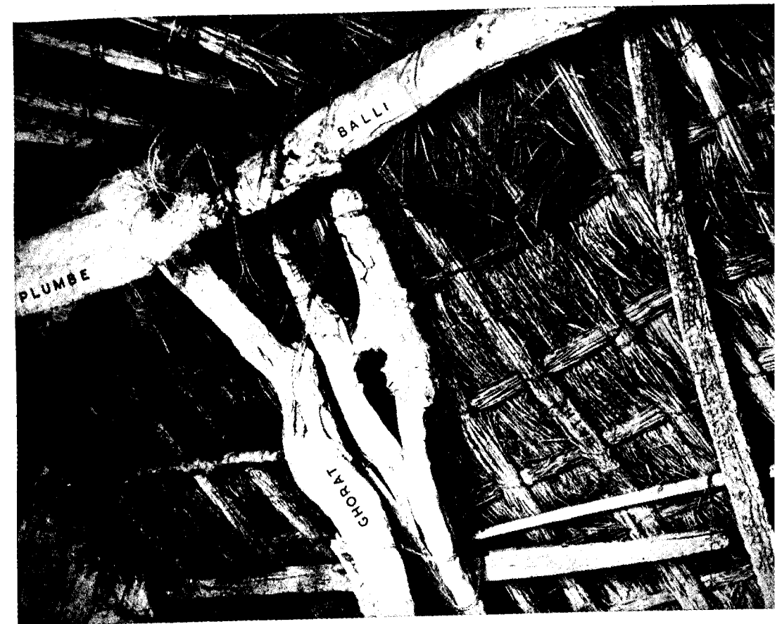
The roof of a chhappar The picture shows the material used in the construction of the roof.
