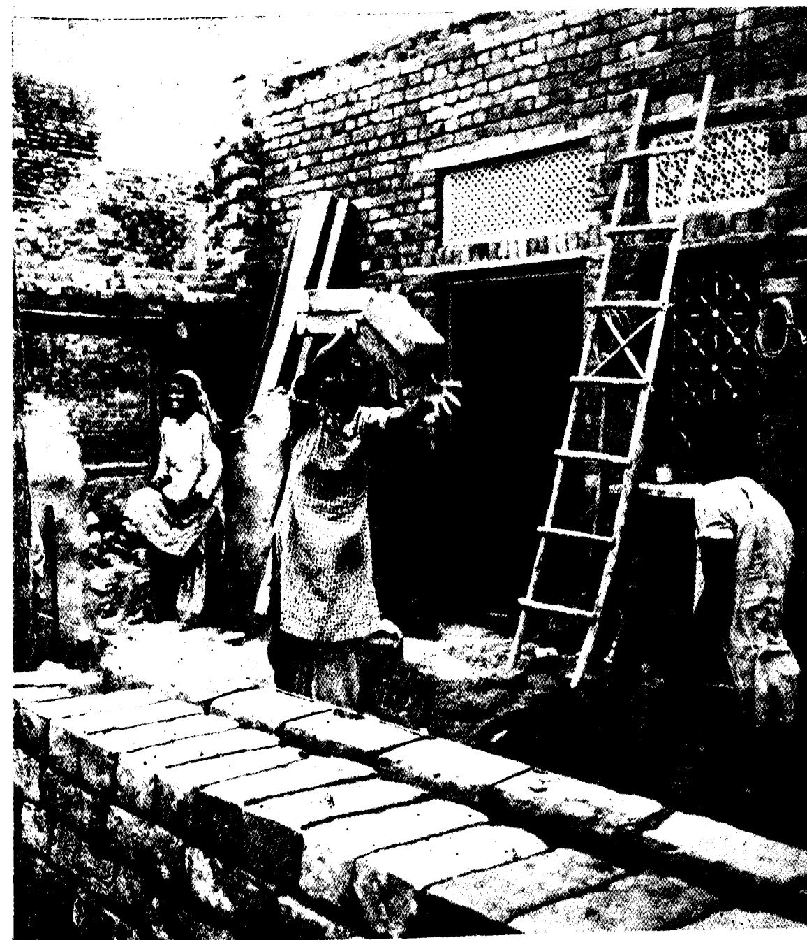
The courtyard of a house being renovated to serve the purpose of extra rooms. Note:—Although it will lead to greater ill ventilation than before, yet the owner is not much worried on that account.
