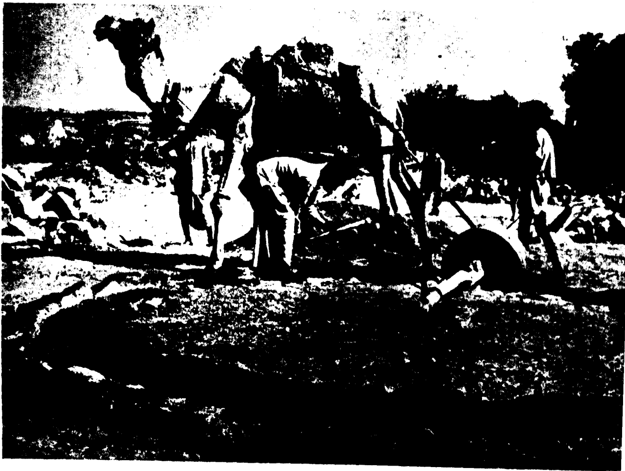
Lime mortar grinding mill--A camel is driving the grinding stone
