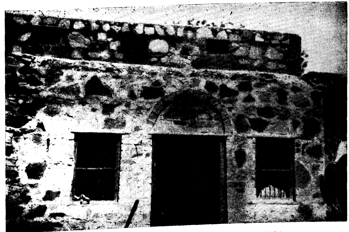
A rubble masonry house in village Yahya Nagar in Mehrauli Block, Delhi.
