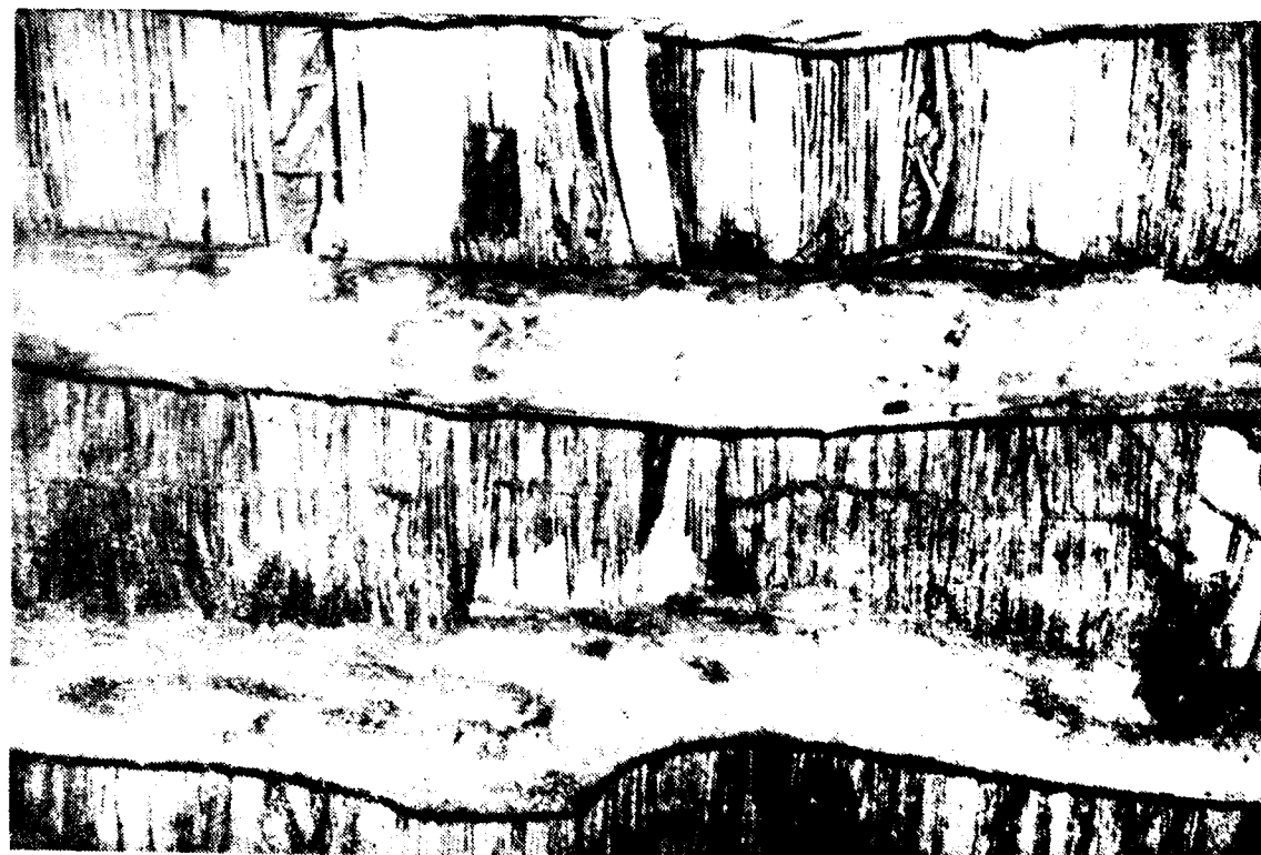
The roof of a mud hut made of joists of 'neem' trees, wheat stalks and thin rope in a Delhi village.
