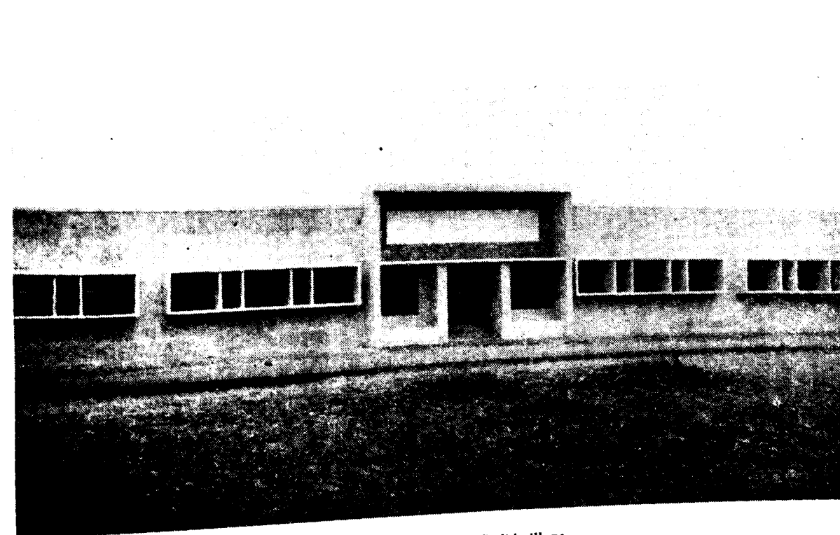
A modern school recently built in a Delhi village.
