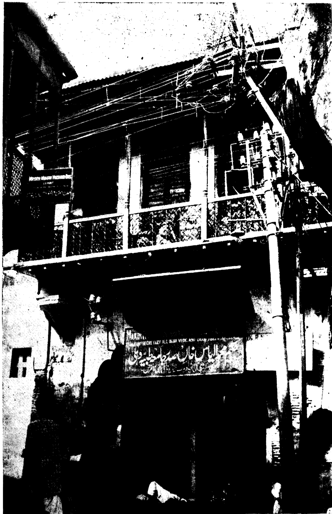
An old building in Balli Maran believed to have been constructed over 90 years back. The building houses a Medical School.
