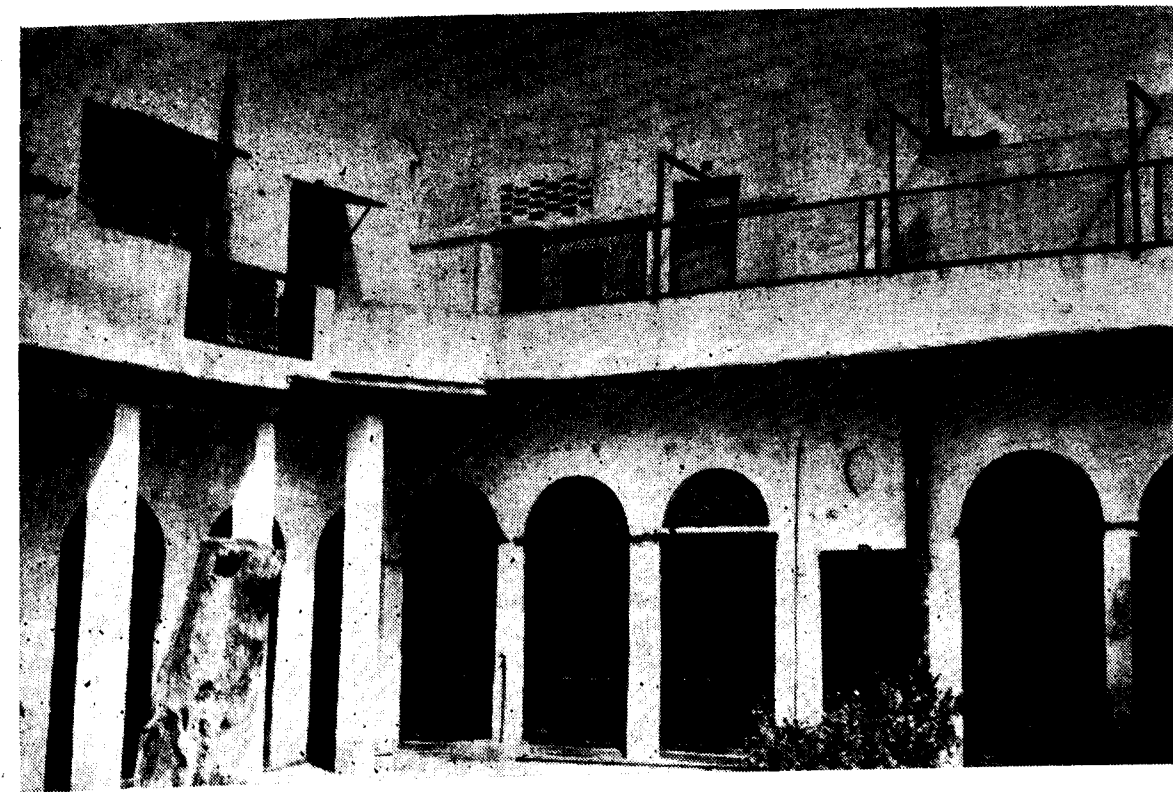
Interior of the Building, where the residential students of the institute stay.
