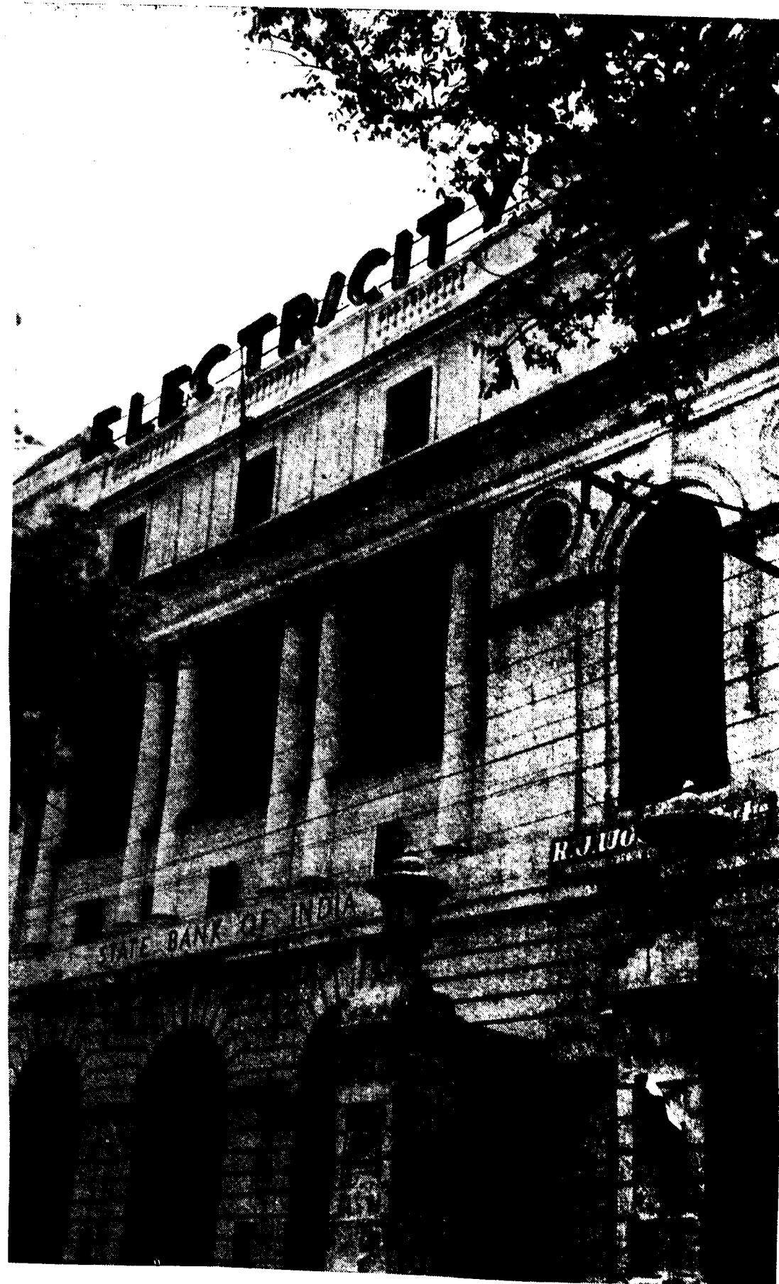
A typical early British construction. The office of the Delhi Electric Supply undertaking and the State Bank of India are at the moment housed in it.
