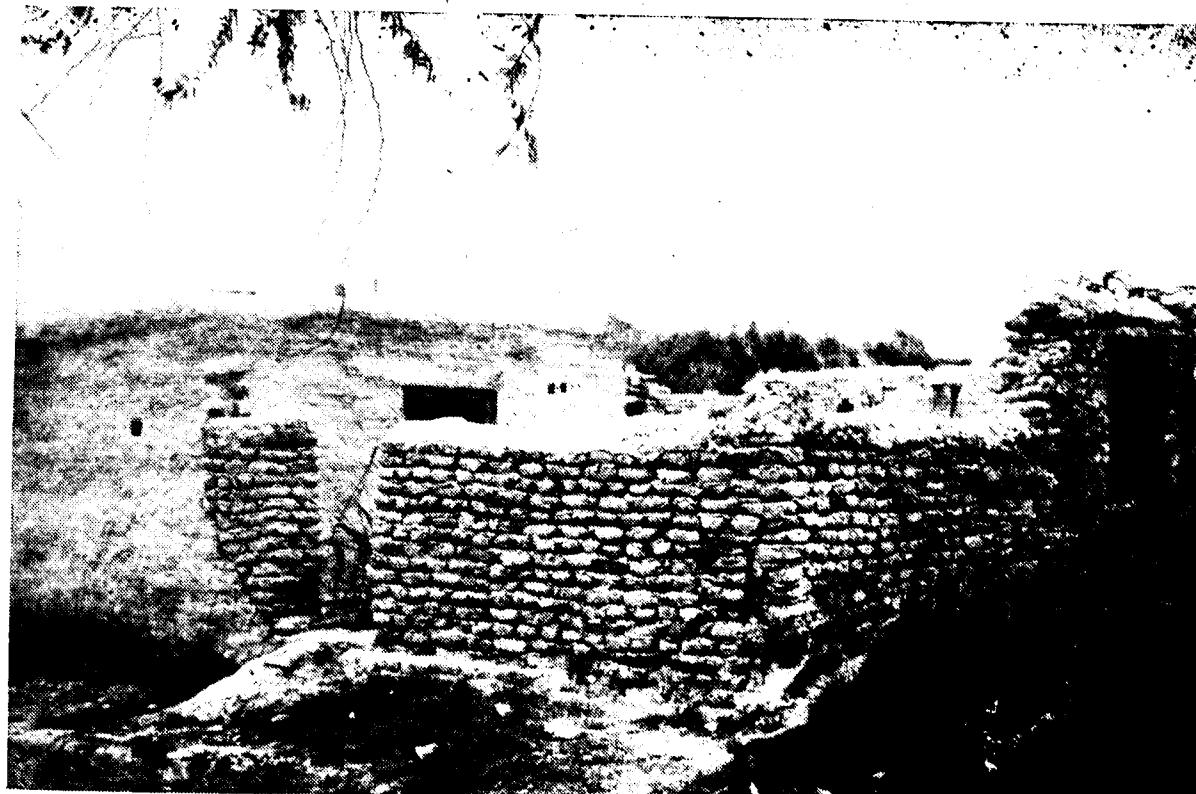
Partly built house with mud bricks.
