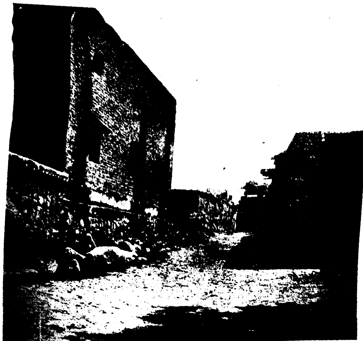
This is a Kuccha street of the village. The building on the left is the village Chaupal.
