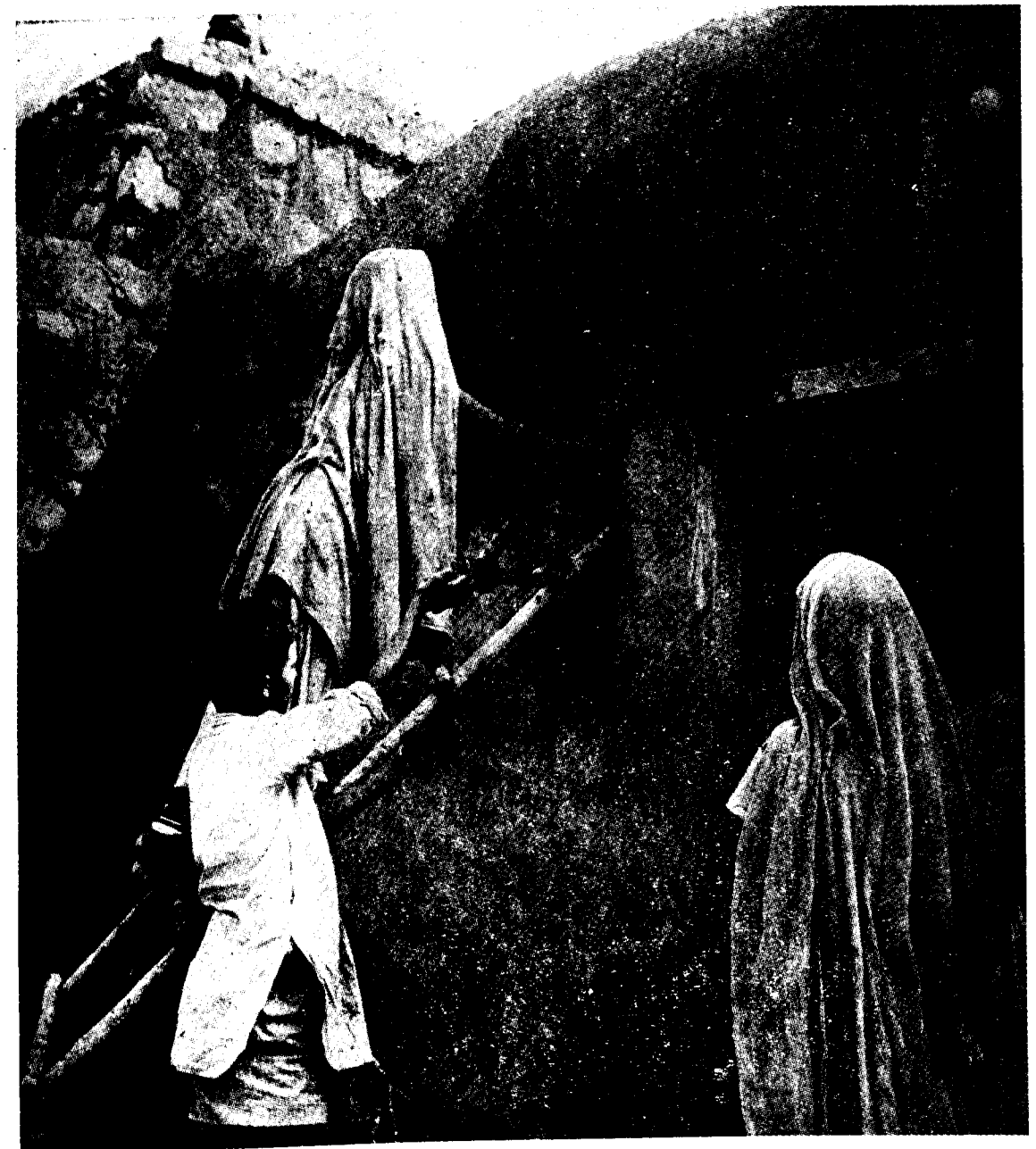
Rains or blazing sun may cause the roof or wall to crack. These cracks are repaired by men and women themselves. The picture above shows a woman and a boy repairing some cracks.
