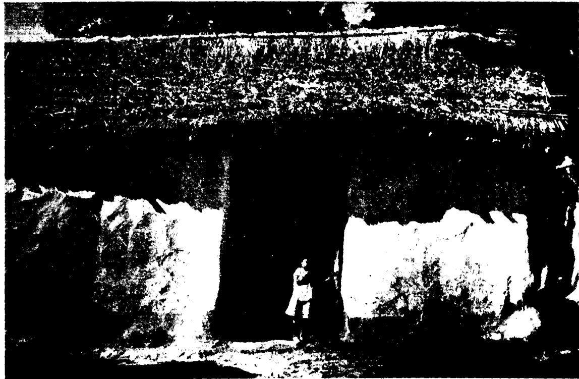
This is a kuccha house, belongs to a CHAMAR. Walls are made of mud and the roof of straw and reeds.
