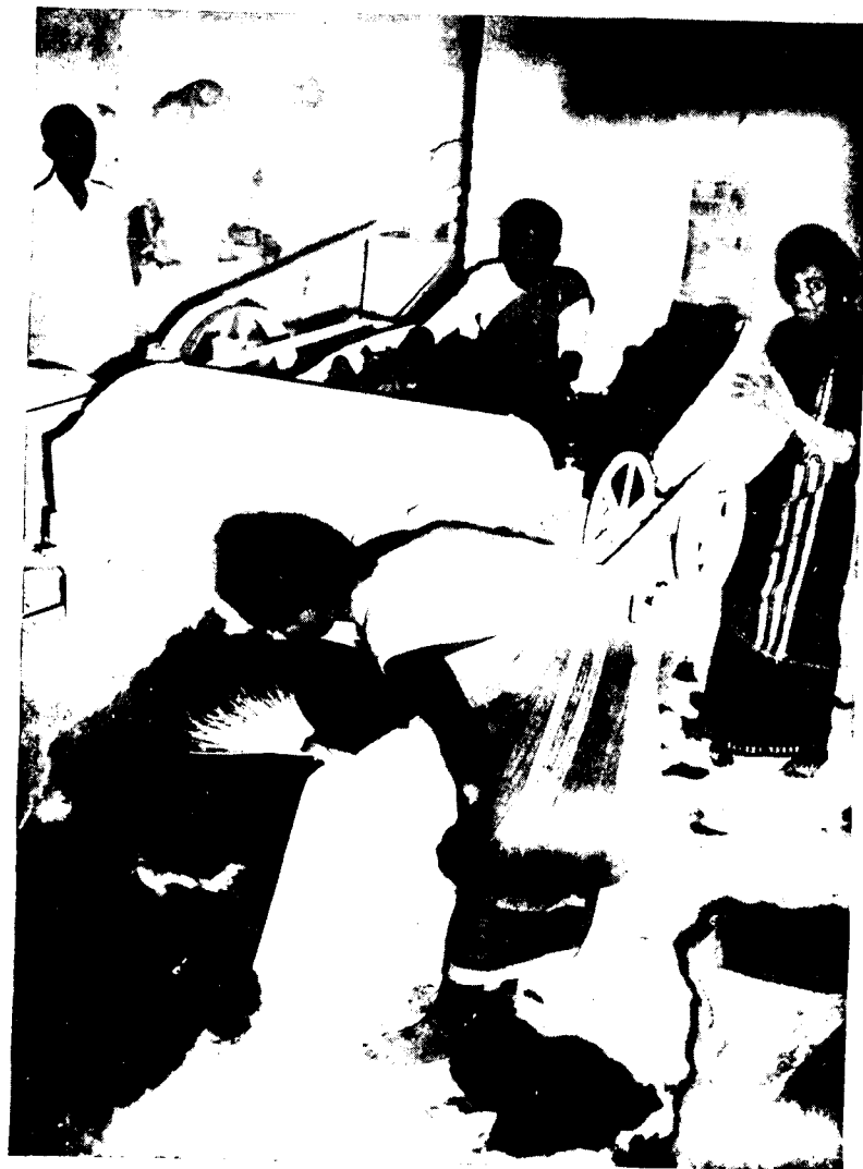
The Nail Drum Carding Machine is set in motion. The lime wool comes into contact with the rolling nails and gets thoroughly teased up.
