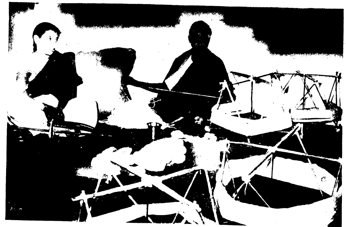
In the house of the woman twister, the cotton yarn of 10 counts for 8 plys is spread into four branches on the two drawing wheels. Note the woman twister holding cotton yarn by her left fingers and drawing the thread by her right.
