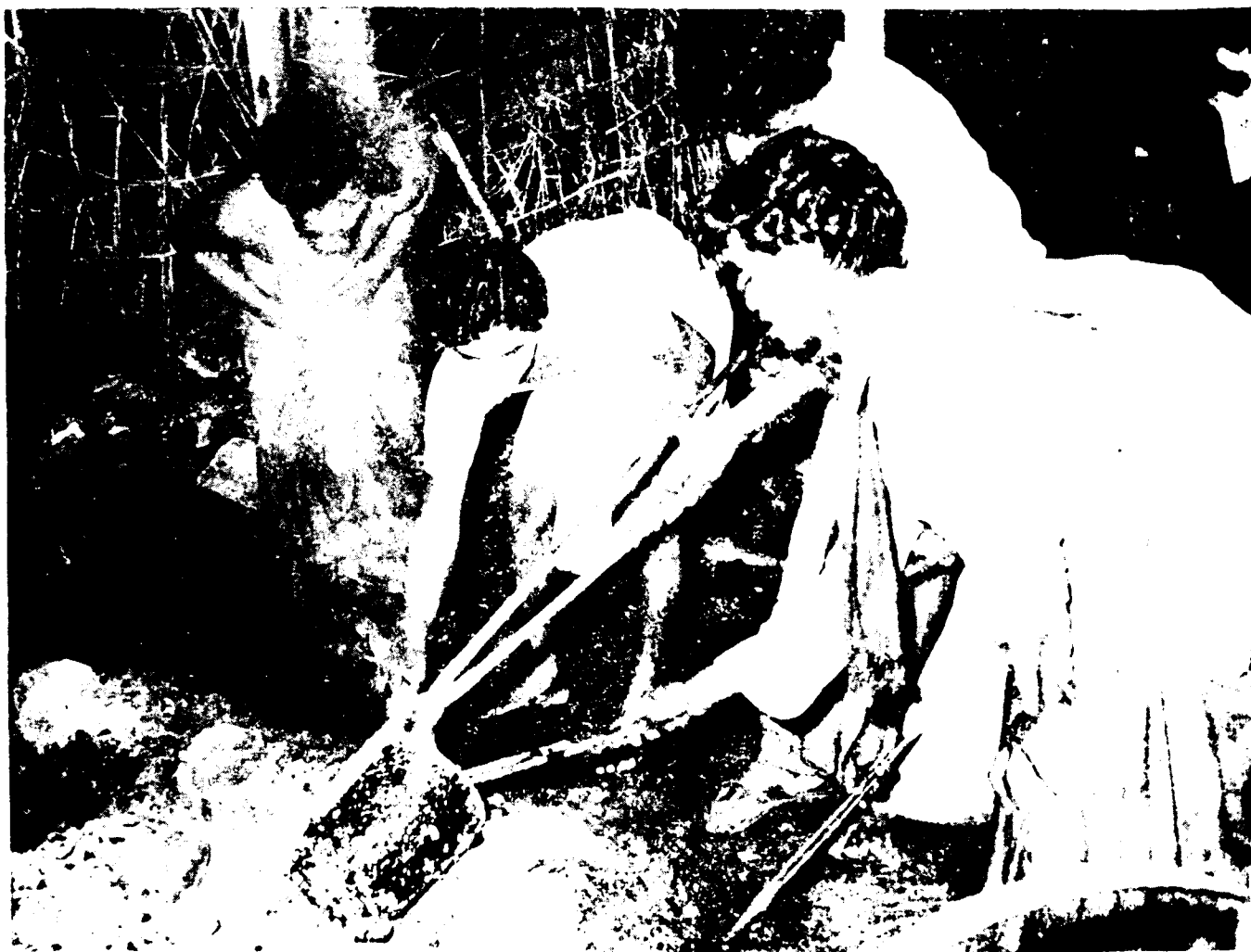
The crucibles are then lifted out of the furnace carefully with the help of the long handled prongs.
