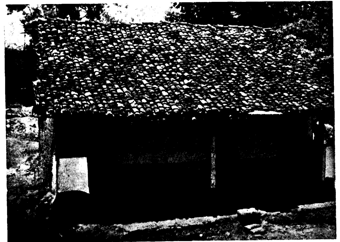
House built of mud walls with country tiled roofing.
