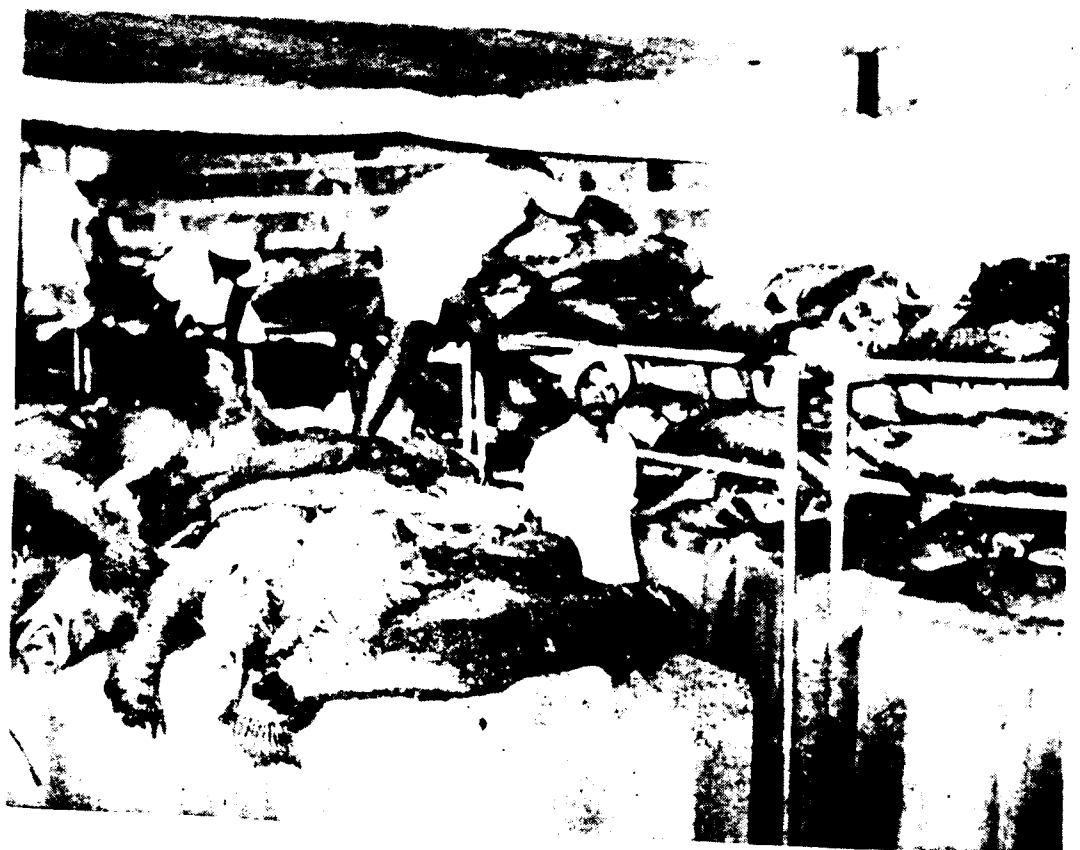
Cold-storage at Veraval
