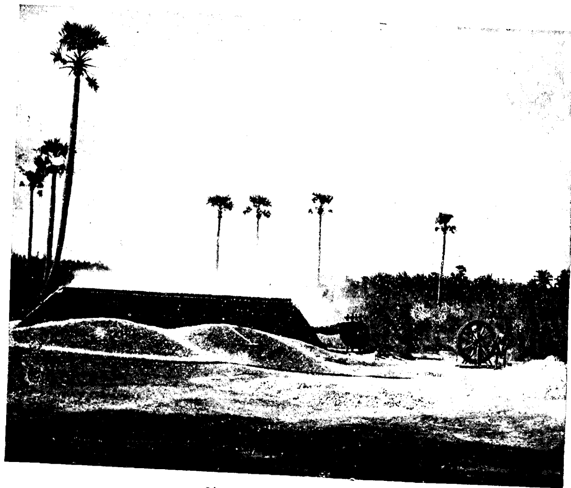
Lime kiln at Sunnambukulam
