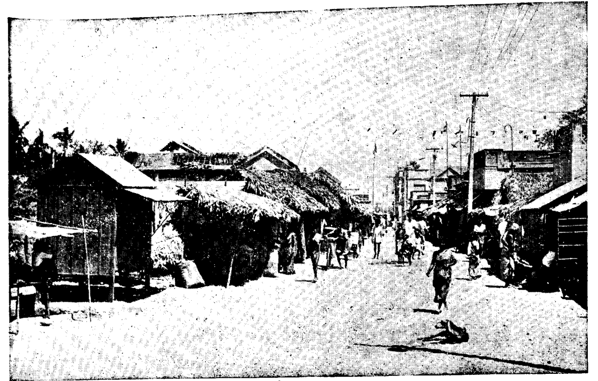
A view of the bazaar street
