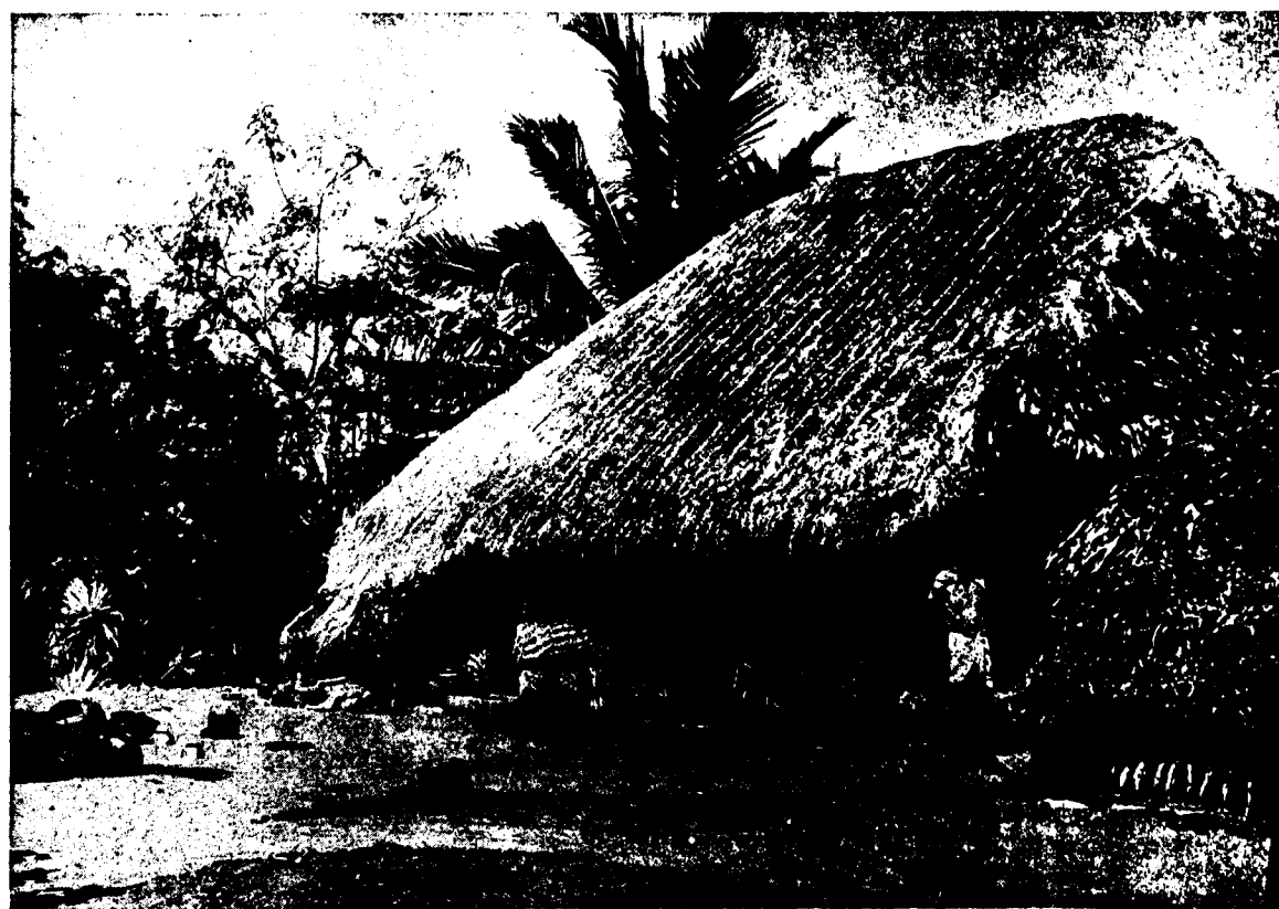
The roof of the hut is reinforced by straw to prevent leakage.
