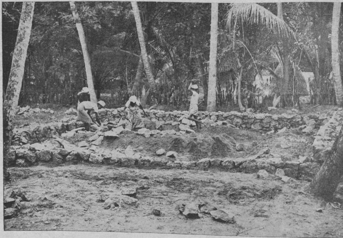
House construction in progress. The foundation is built of granite stones and random rubbles.
