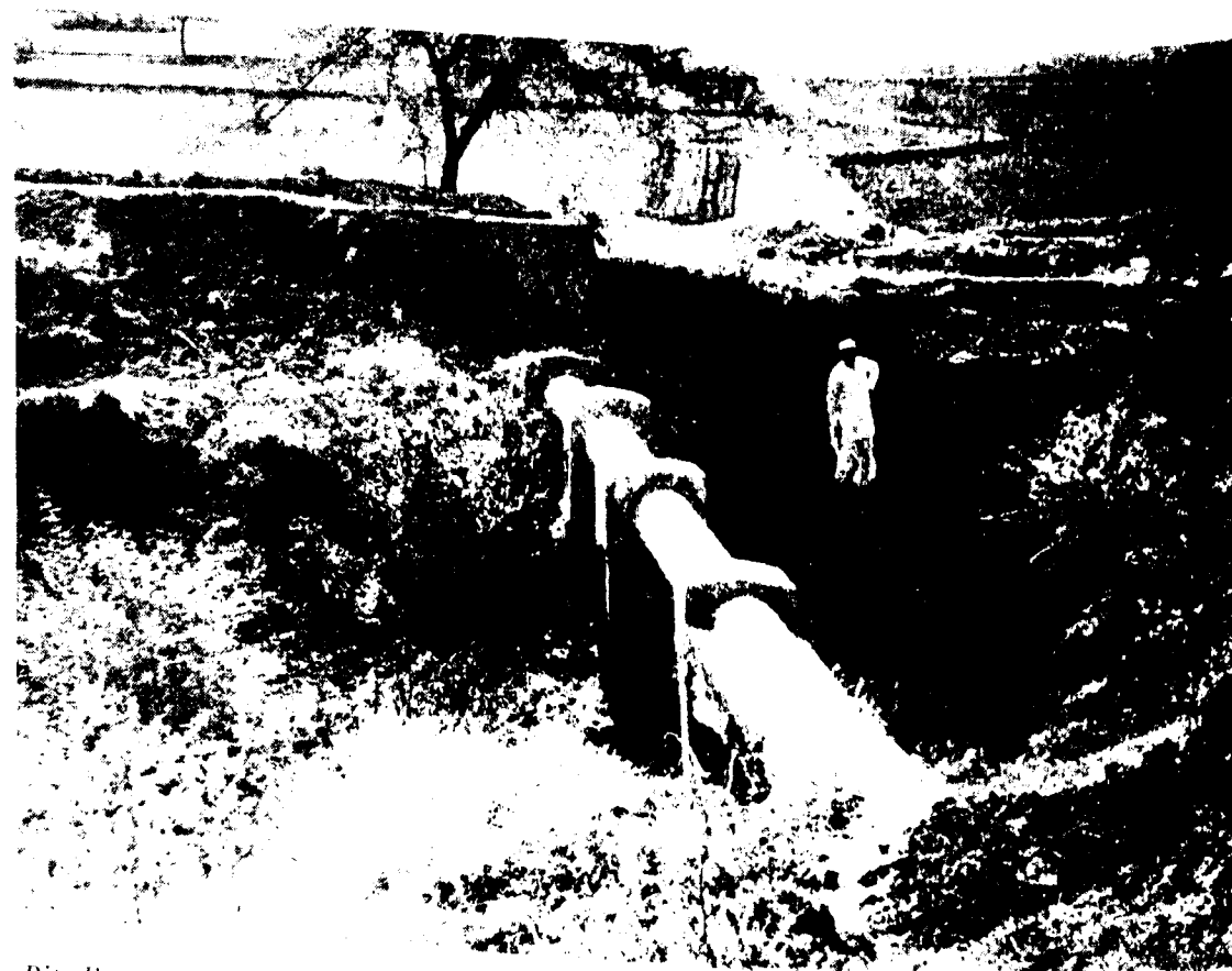
Pipe line of the Mahi canal distributary passing through the village without any benefit to its cultivators
