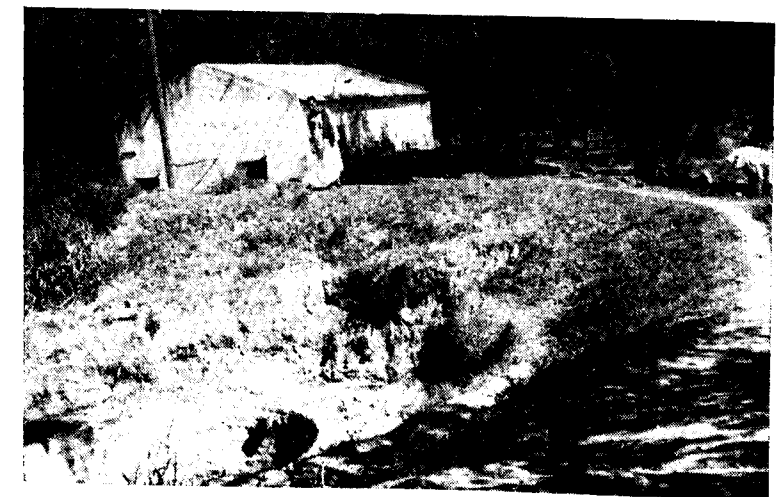
Photo 6. House for the farm pump set
