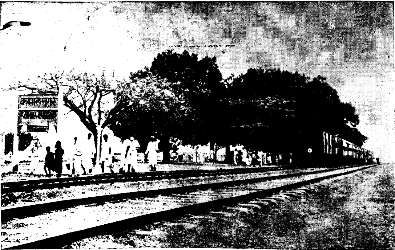
1 THE RAILWAY STATION—KAMALNAGAR
