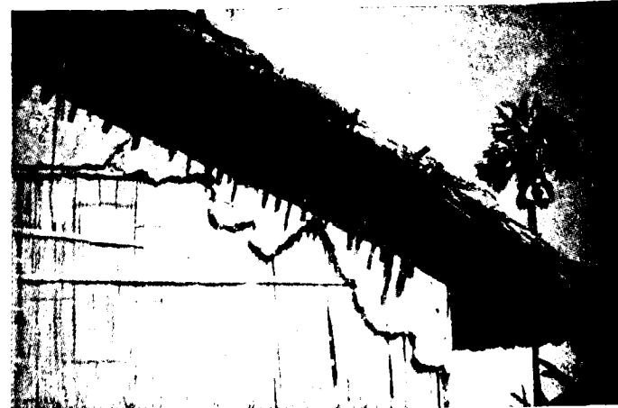
38. A house wall with part of mud covering worn off
