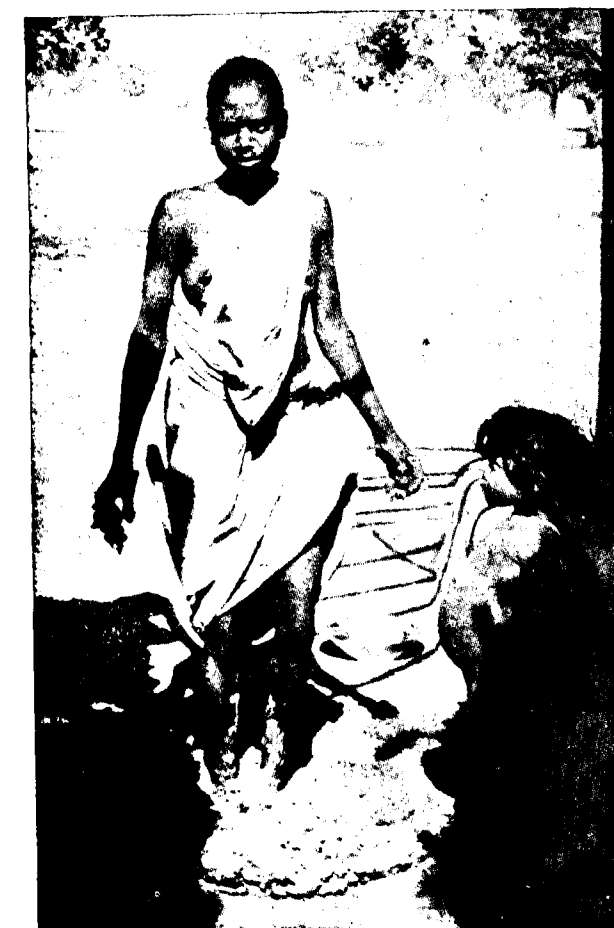
66. Preparing the mixture for house repairs
