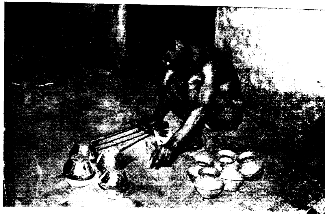
Filing is usually done after the various moulded parts of a utensil have been soldered. Sometimes a little filing is necessary before soldering, too. —Photo by courtesy, B. C. Industries
