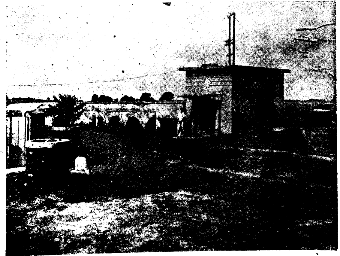
The Pumping Station
