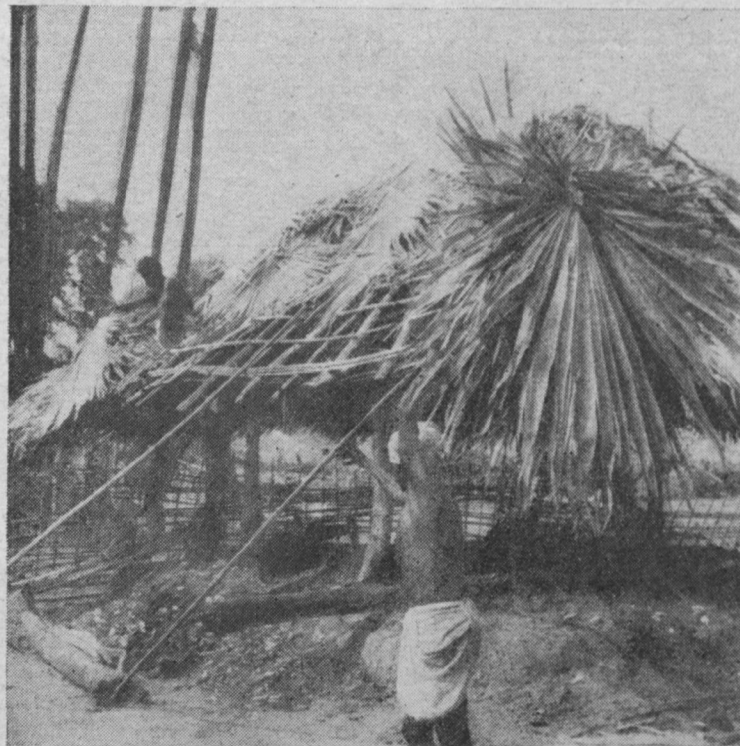
Fig. 9—Process of covering the roof. (Chapter II—Para 30)
