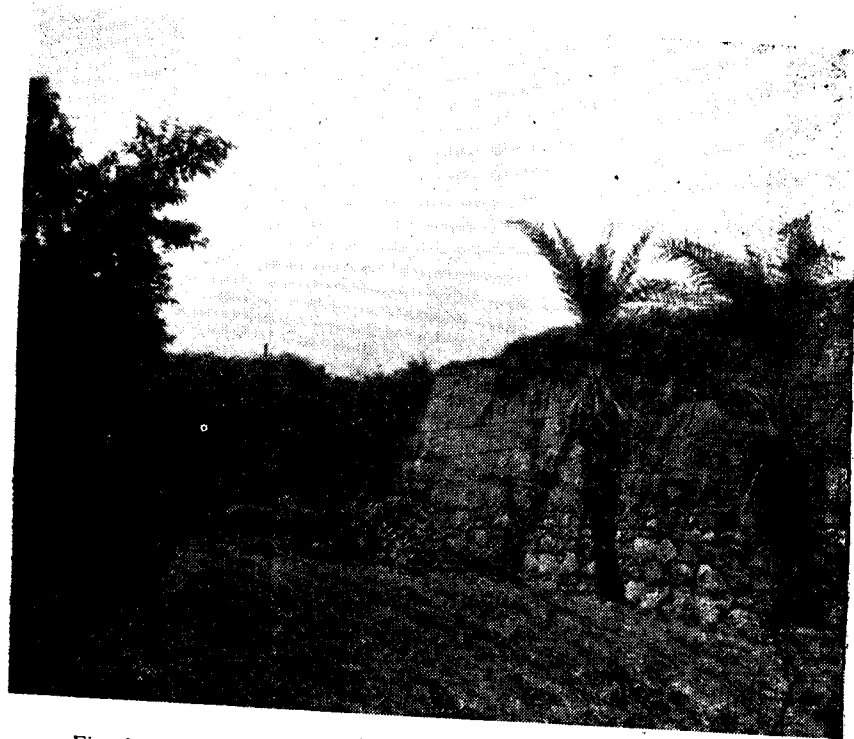
Fig. 2 Guraju—A dilapidated monument. ( Chapter I - Para 19 )
