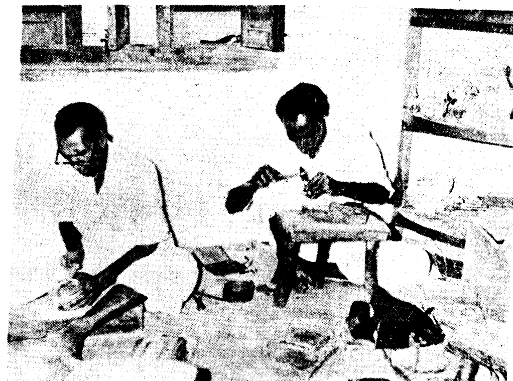
Plate 21. Smoothing a round article with files and engraving a box.
