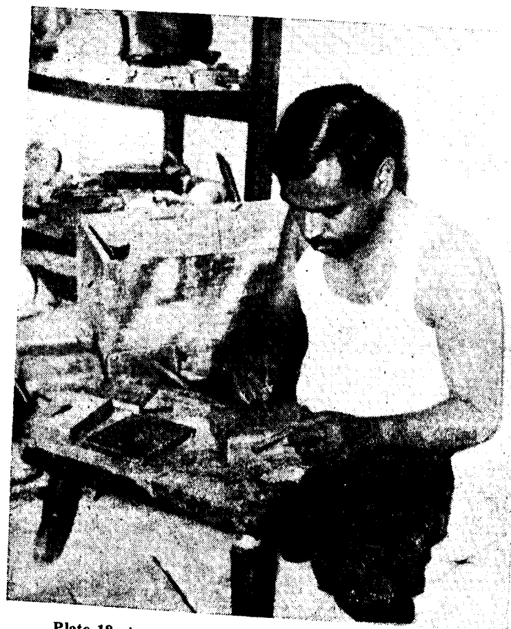
Plate 18. A worker marking designs with a sharp kalam .
