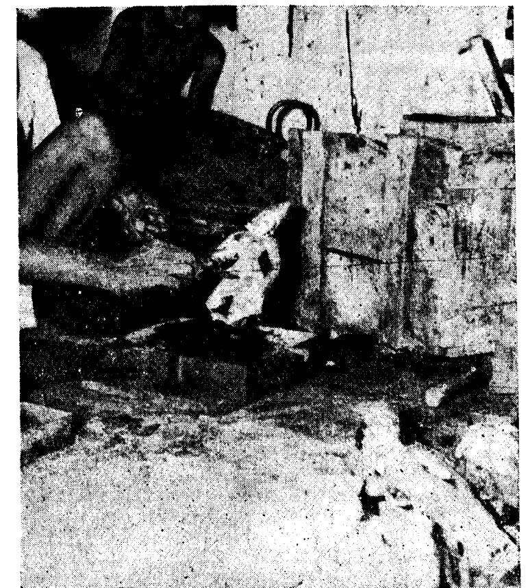
Plate 13. Cast image of Padmapani Buddha taken out from clay mould.
