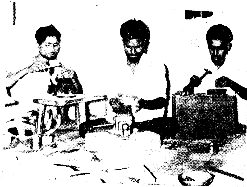
Plate 22. Chasing on different types of articles.
