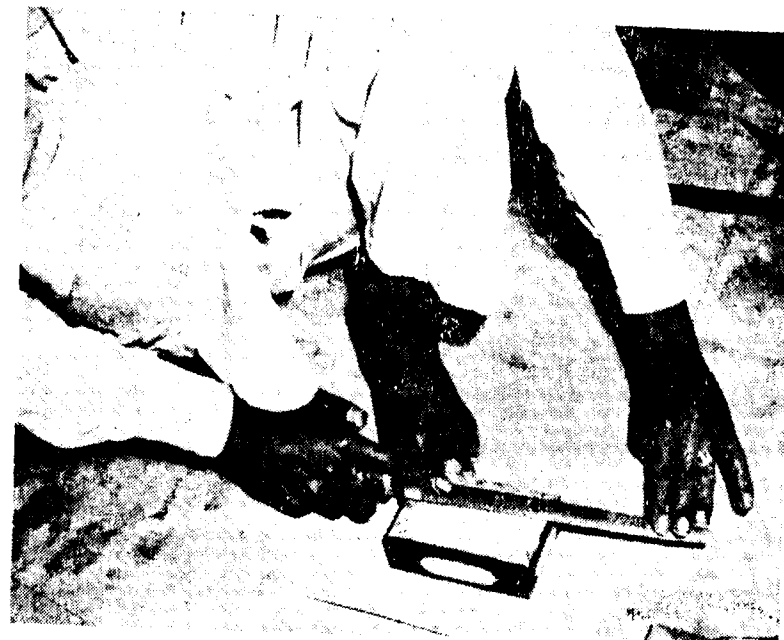
Plate 26. Filing silver embedded surface for common level.
