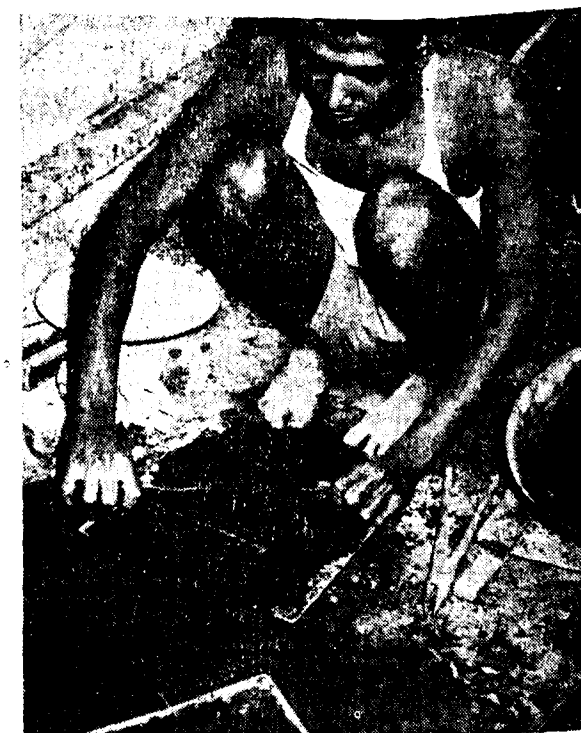
Plate 4. Darza box filled with clay.
