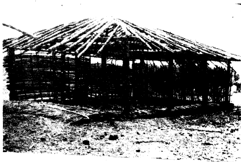
Fig. 5—A house under construction. (Chapter II - Para 52)
