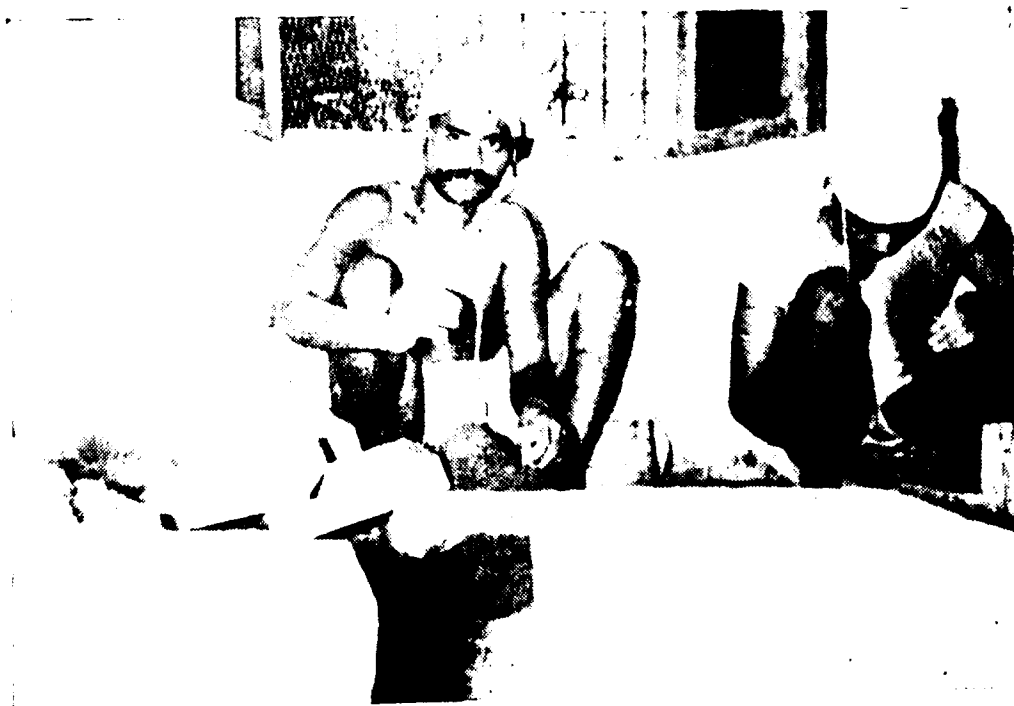
Plate 4. The workers at the process of making moulds with earth and wooden frames.
