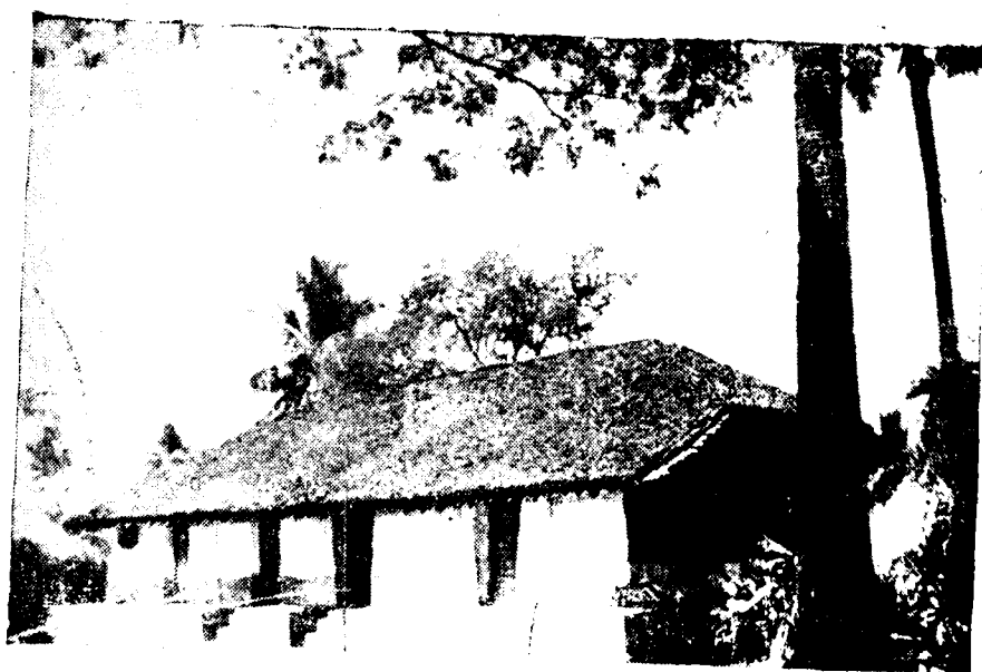
Plate 16. House type of a well-to-do Agnikulakshatriya family in Ponnappalle area.
