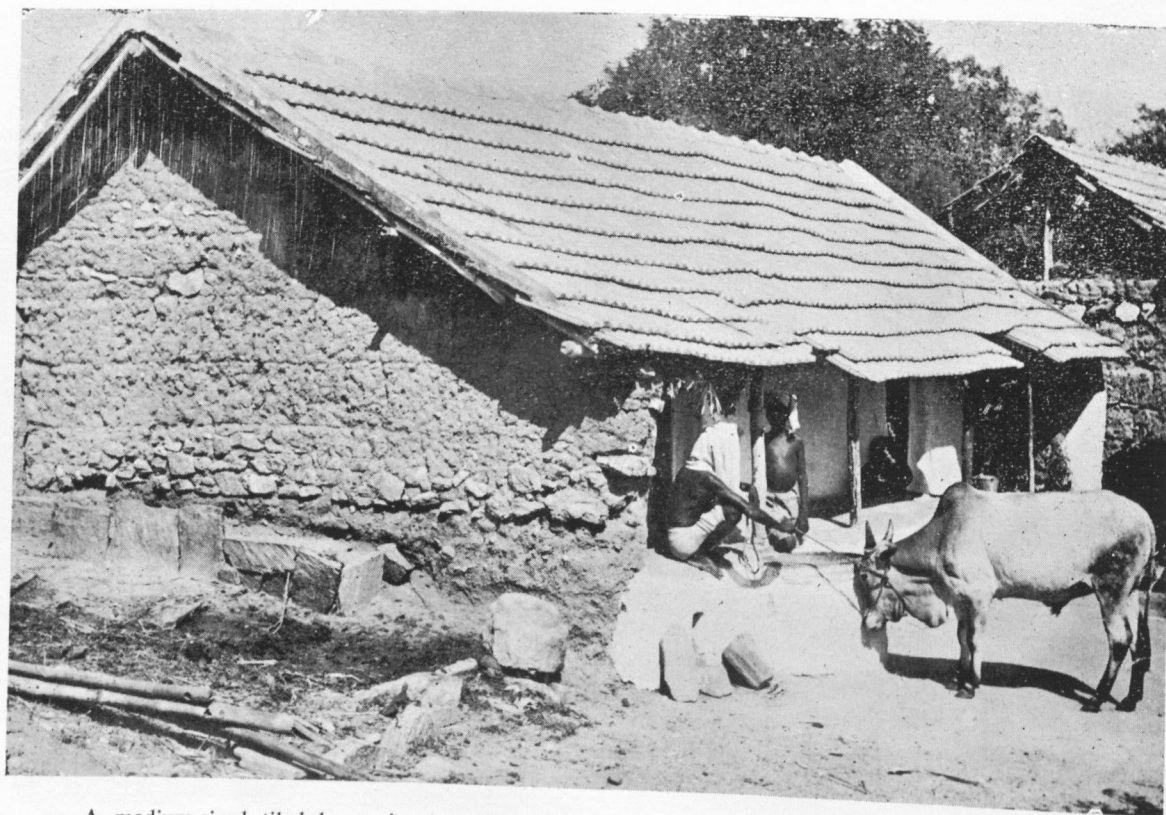
A medium-sized tiled house in the village. Note the walls built of random rubble and mud,
