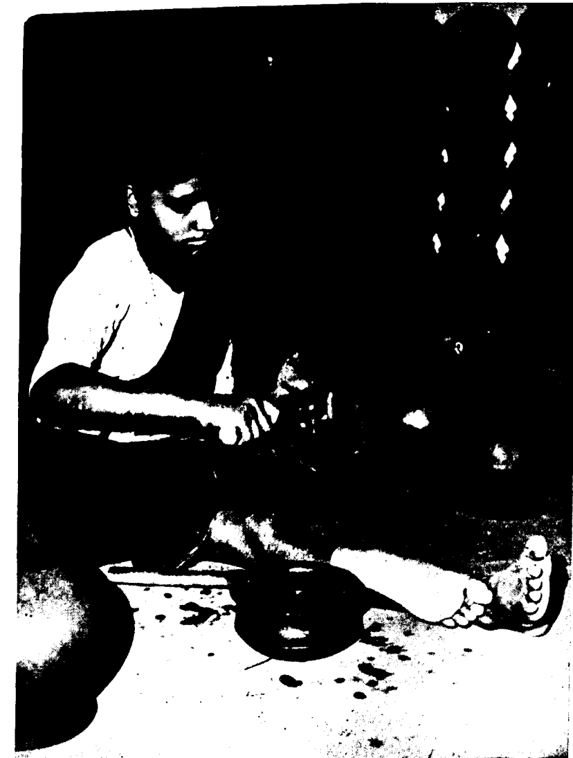
A woman rotates the pot by her left hand and slowly and steadily beats the bottom of the pot which makes the clay spread out on all directions, and thereby the texture of the pot becomes thin.
