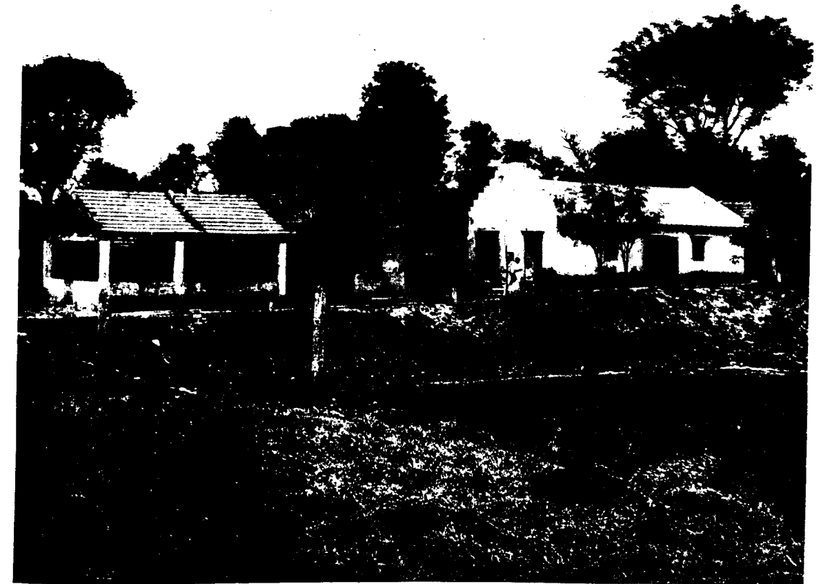
The premises of Karigiri Cooperative Society and the two huge un-utilised Kilns built by government assistance which demands high cost of operation to handle it
