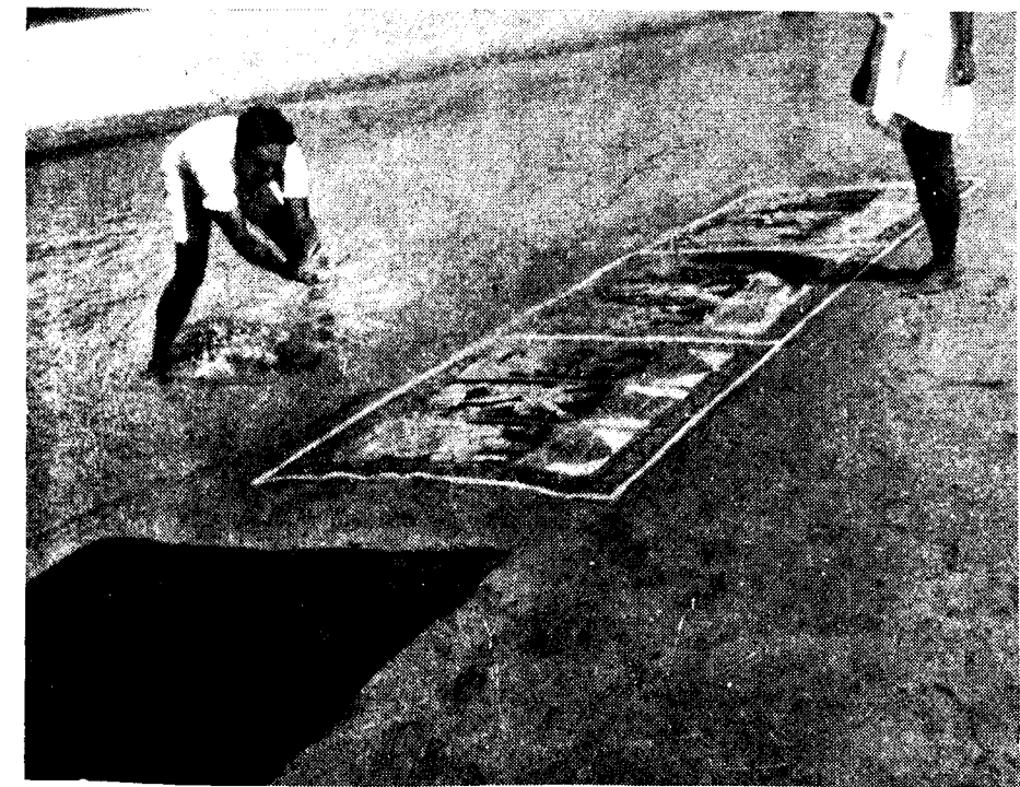
Plate 9. The dyed cloth spread on the river bed for bleaching is constantly sprinkled with water.
