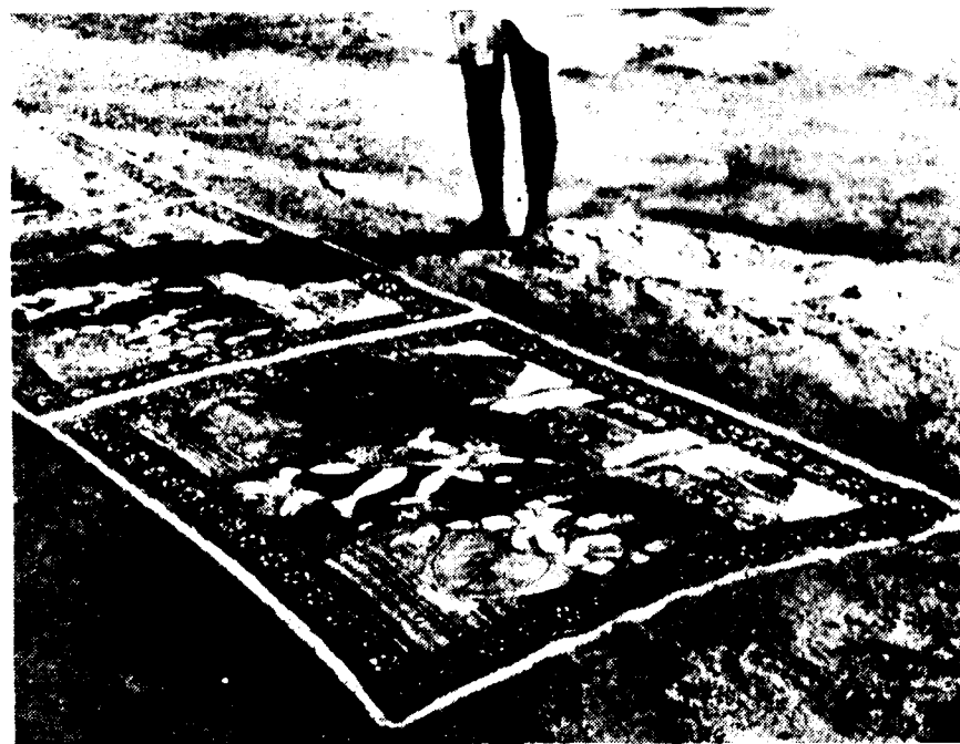
Plate 11. Dyed cloth spread on the river bed at the end of the bleaching process. [It may be noticed that areas to which alum solution had been applied have taken deep red colour and other areas such as the body of the figures, etc., have been bleached into pure white.]
