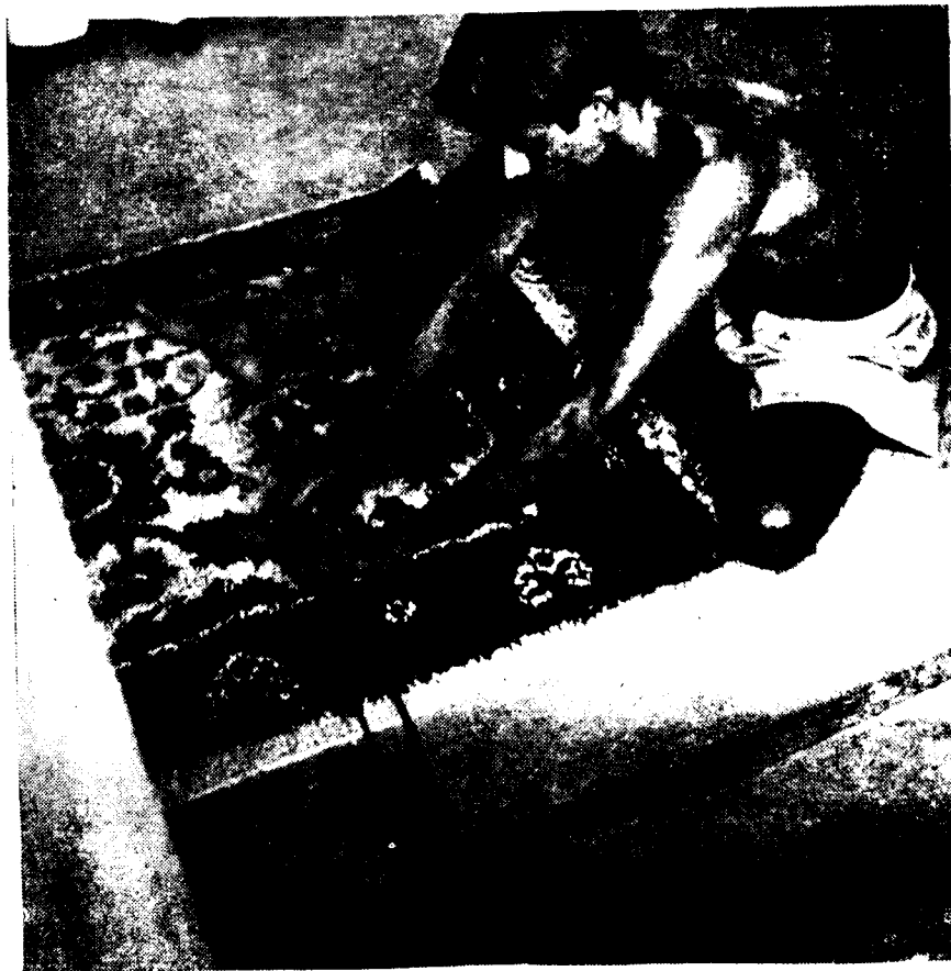
Plate 5. Carpet being cut to level with finishing shears.
