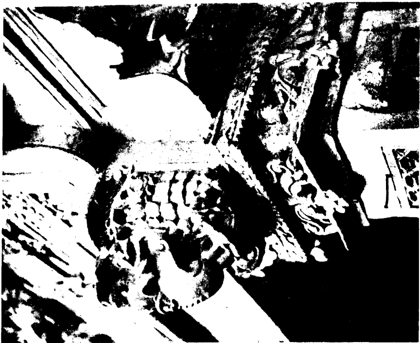
'Sundhiya' (Elephant trunk) on the capital which eliminates the use of a bracket
