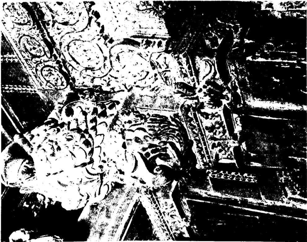
'Sundhiya' (Elephant trunk) on the capital which eliminates the use of a bracket
