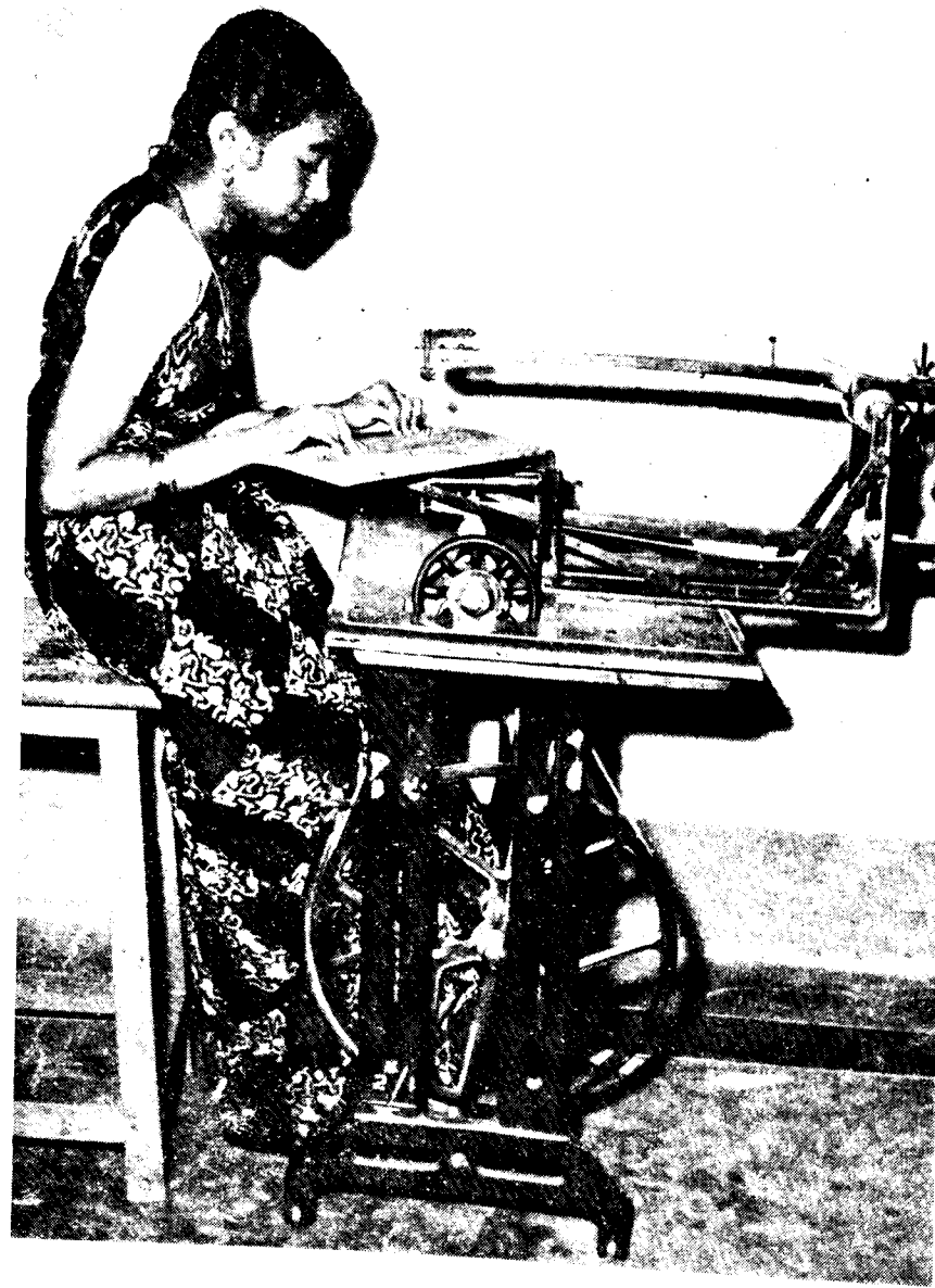
The operation of fret machine is similar to that of a sewing machine.
