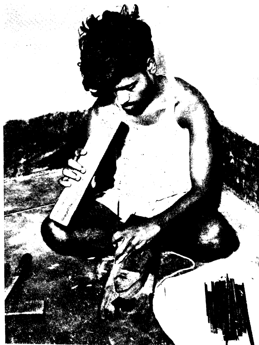
Wood is reduced to shape. Chisels and mallet are used.
