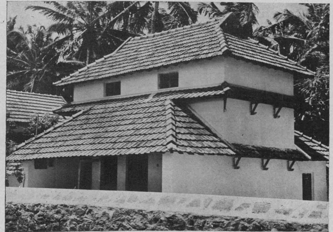
The tiled house of a prosperous Sambavar in the village.
