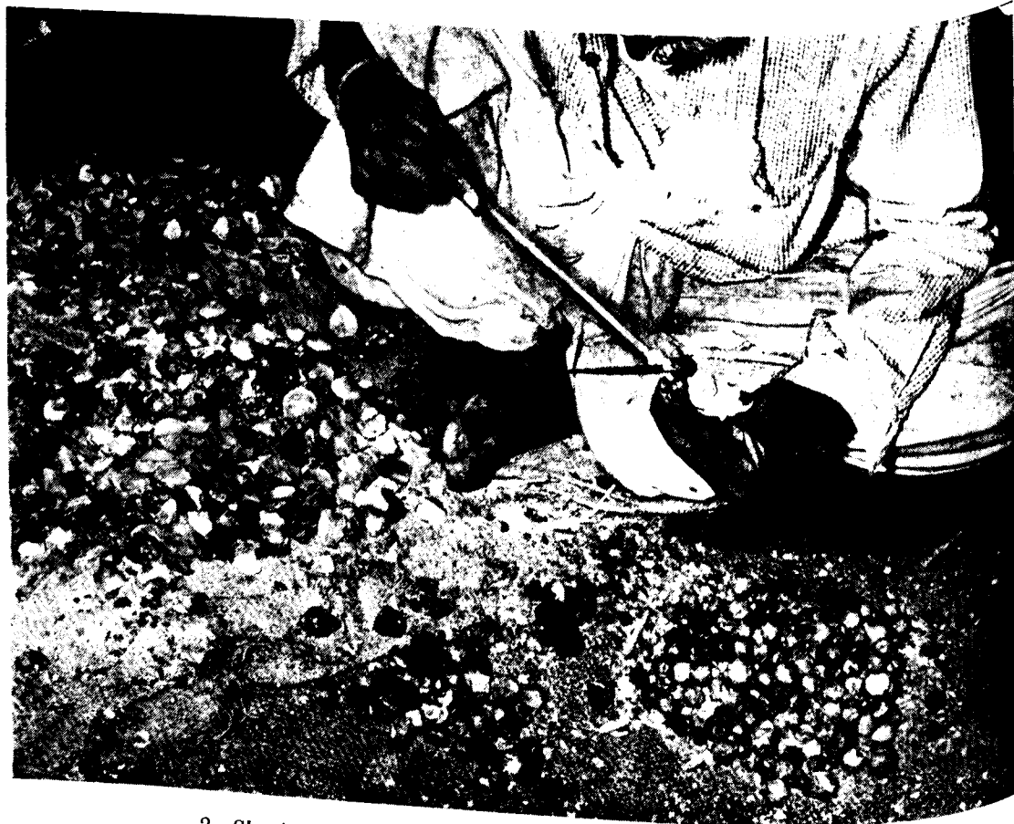
2. Shaping the stone with nail-shaped hammer for ro
