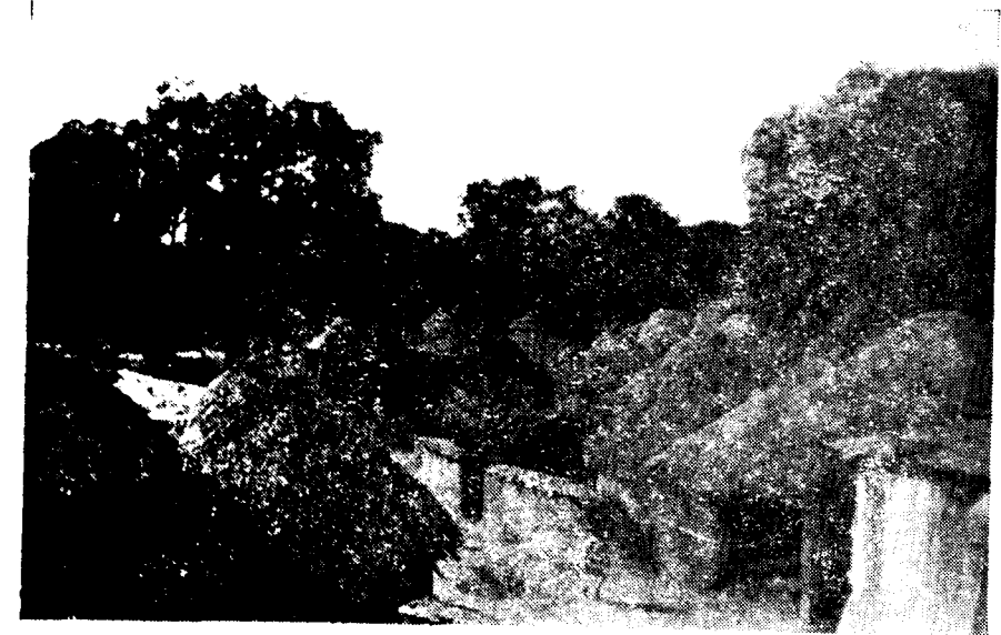
Photo No. 11 Typical round huts mud walled and thatch roofed in Cuddapah and Chittoor districts.
