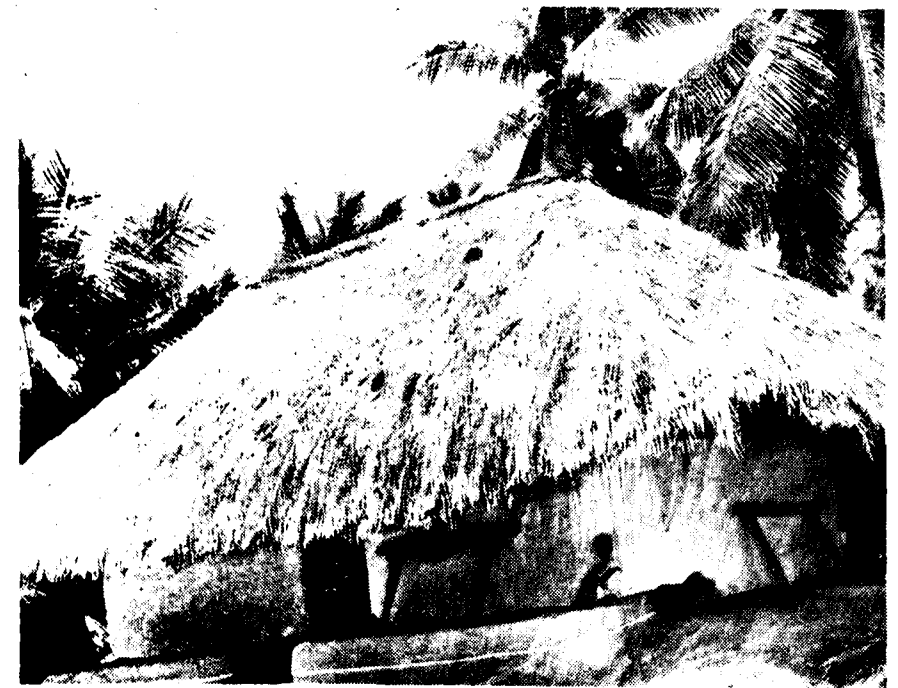
Photo No. 6 A typical dwelling in the delta area of East Godavari district with coconut leaf thatch and mud walls.
