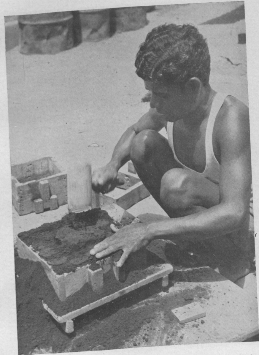
The moulder fits a wooden runner over the metal pattern mould so that it connects with the mouth and cavity in the bottom box. With his right hand he then fills the top box up with vandal sand to the top of the runner and with a wooden mallet he rams the sand flush with its upper edges.
