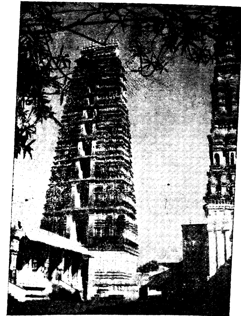
Fig. 30 Galigopuram -entrance tower of Sri Lakshminarasimhaswamy's temple at Mangalagiri-it is 125 feet in height with 11 storeys. It is one of the highest gopurams in South India ( Chapter V, para 28 )
