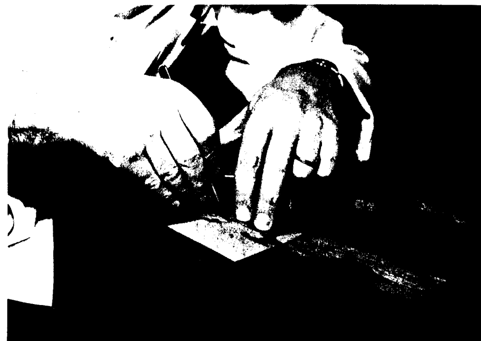
PLATE 4. Cutting repair material and shape of repair area.
