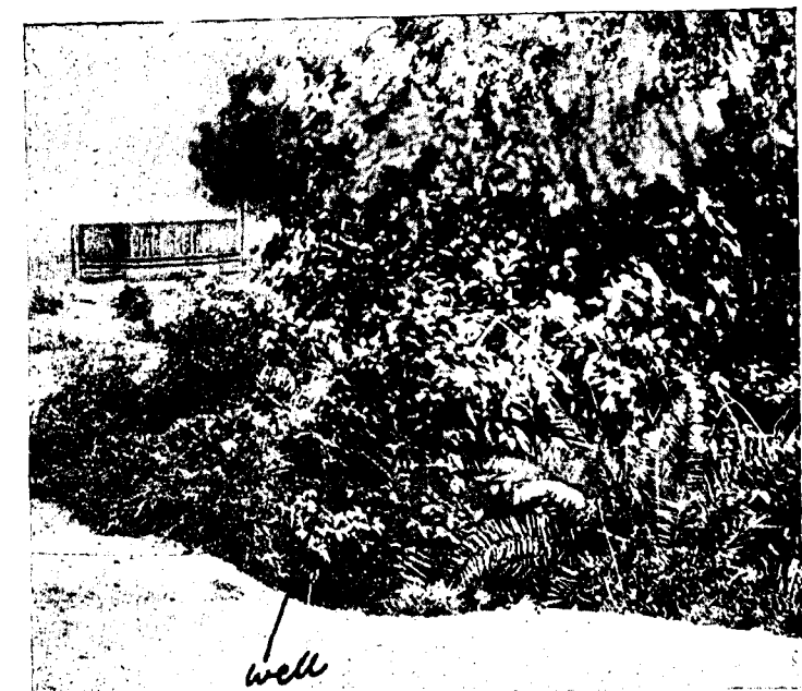
The Mount of Sārangadhara. In the foreground is the well underneath the cluster of trees into which Chitrāngi is said to have been thrown. In the back ground is the temple of Sārangadhara now under construction.
