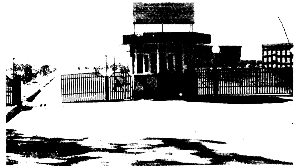
(i) Entrance Gate
