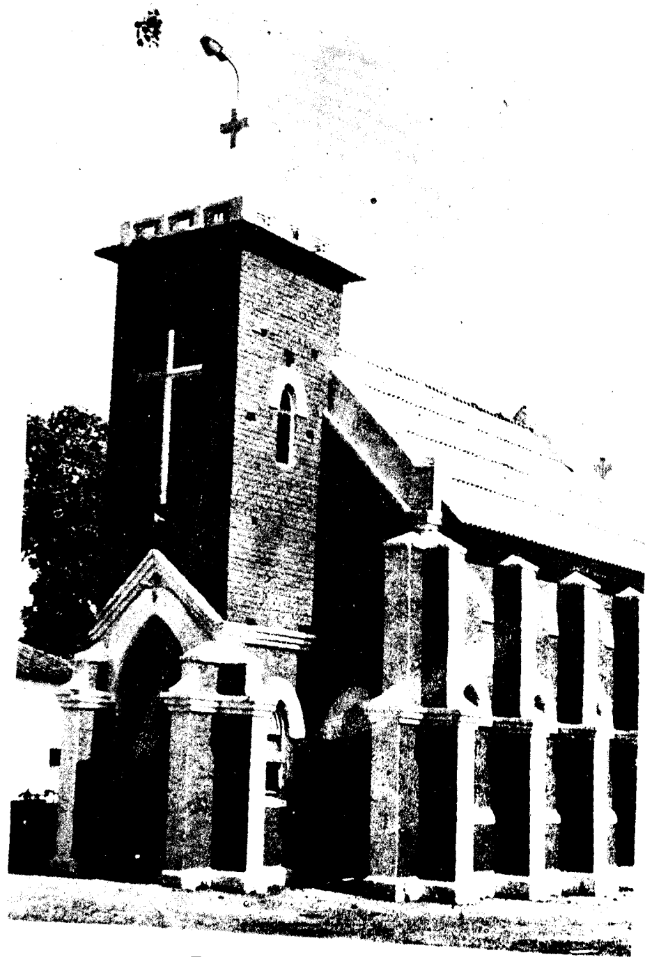
The Methodist Church, Balaghat
