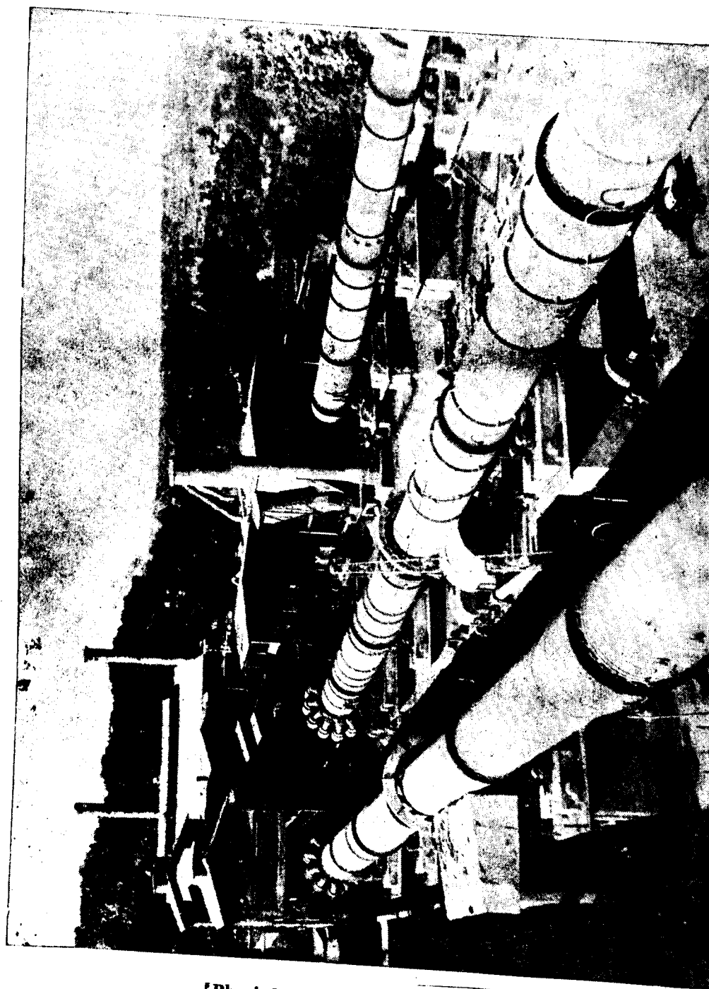
Bhupindra Cement Works, Surajpur
