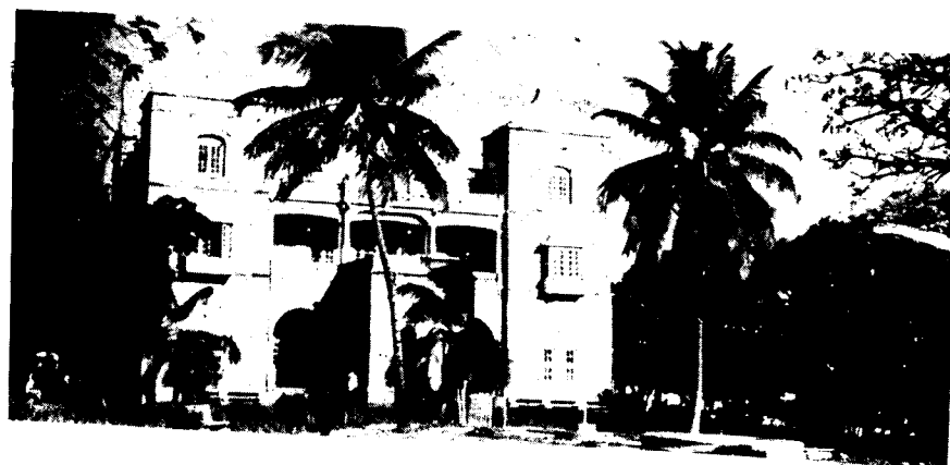
The Hubli-Dharwad Corporation Office, Dharwad
