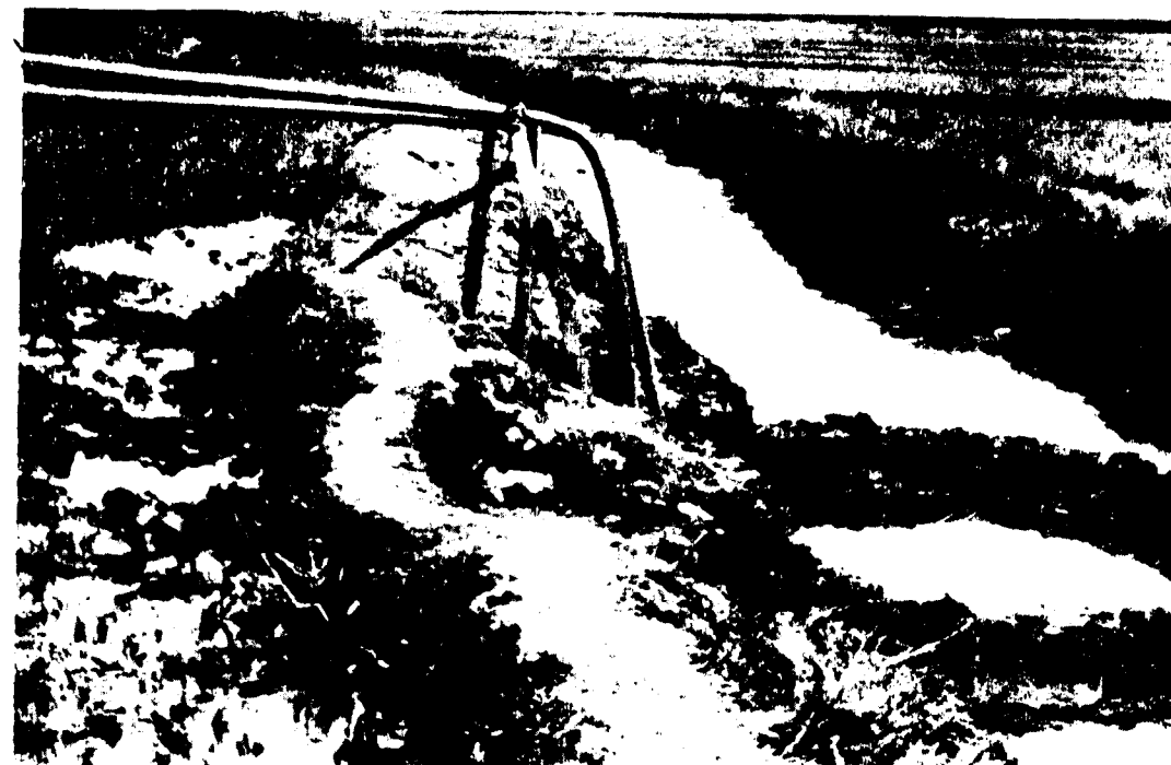
A water pipe line for irrigation
