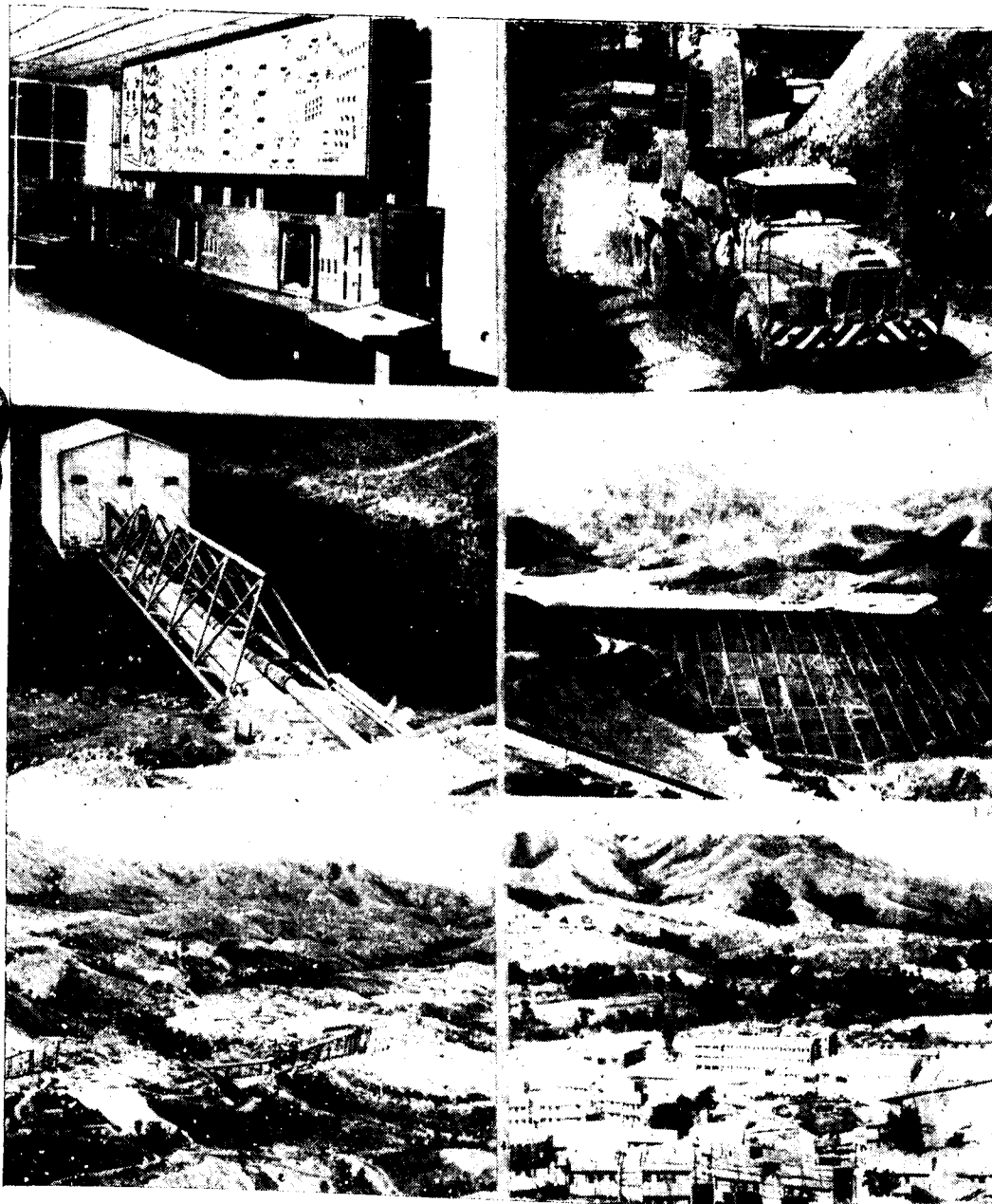
(8) Various stages of completion of the work
