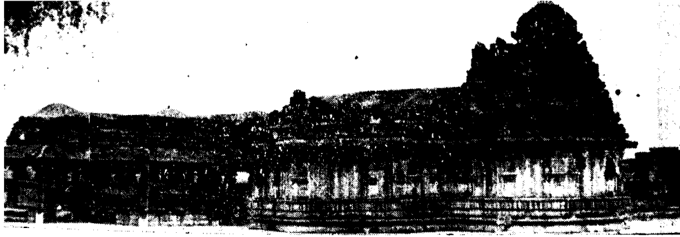
The Amritheshwara temple, an exquisite Hoysala structure at Amrithapura (near Tarikere)
