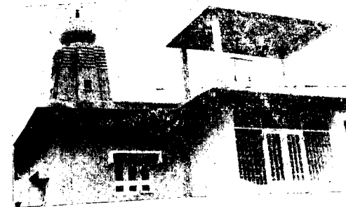
Unfinished Radhakrishna temple at Malleshwara (kudramukh)
