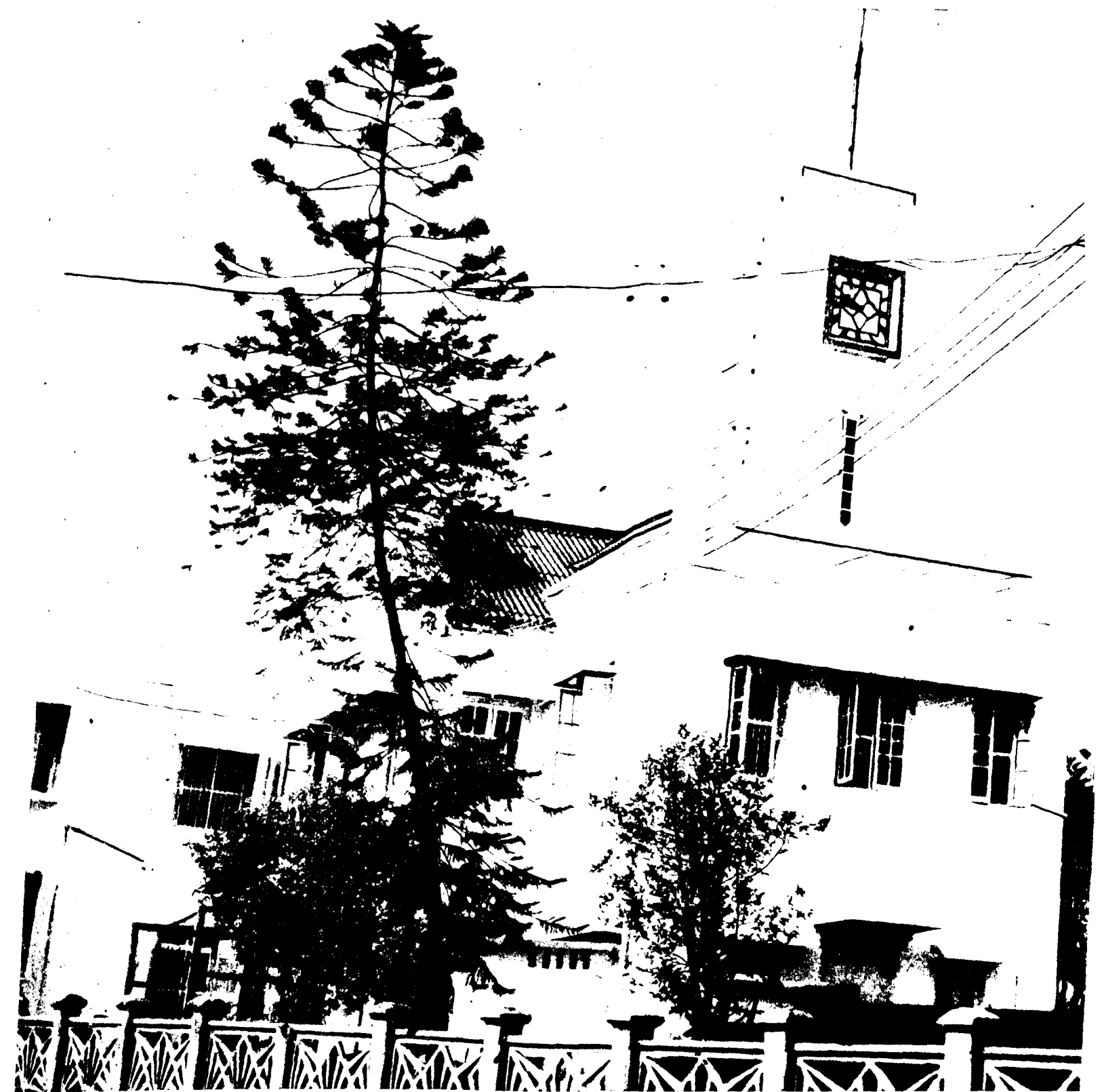
KOTTAYAM MUNICIPAL OFFICE
